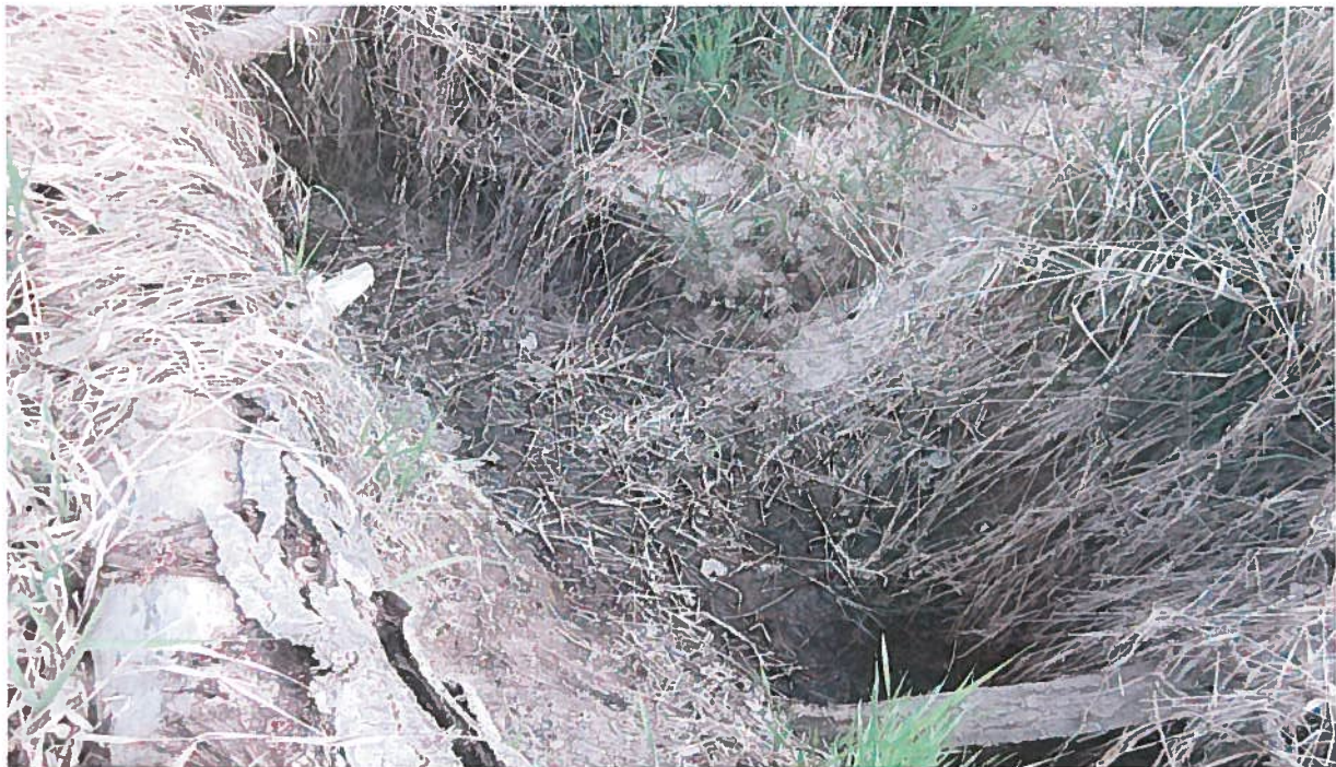
Diversion ditch to the pond.
