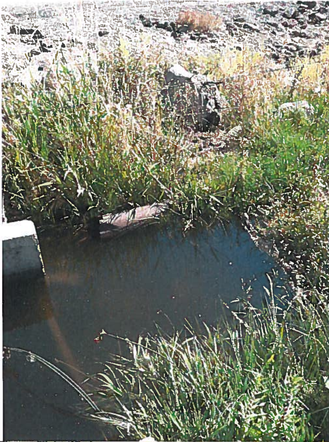
ponded area at PD
