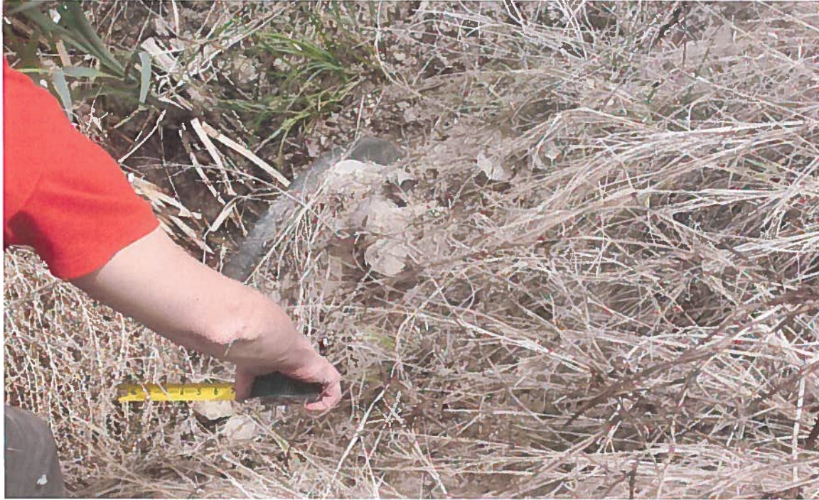
The 22" diameter culvert on the north side of Beacon Light Rd. Little Gulch Creek flows under the road to the applicant's pond.
