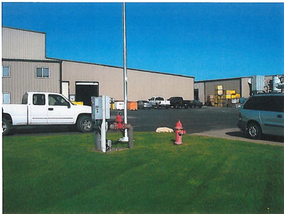
63-31632 Exam 8/24/2012: Portion of POU (Allied Seed facility) with well and fire hydrant in foreground facing west/northwest.
