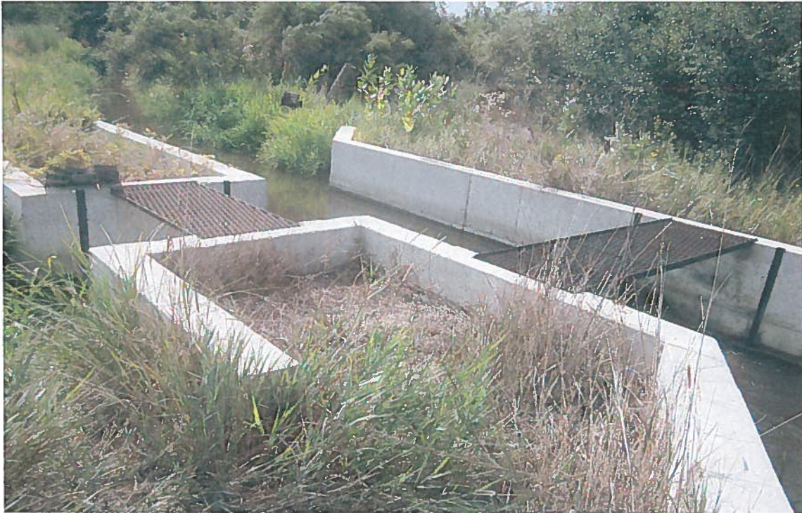
Main inlet on irrigation ditch. Looking southeast. Grate seen left is over the ditch that carries water north to structure # 2, then into cell # 1.
