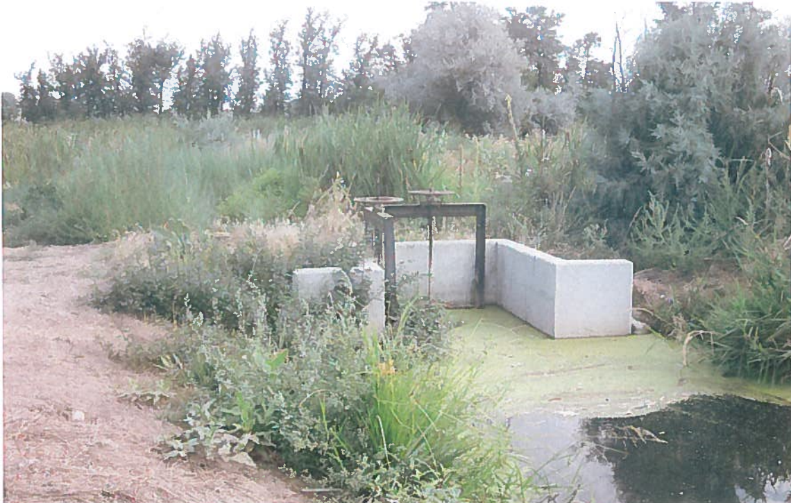
Looking north at structure # 2 that carries water under the dirt road to cell # 1 – west.
