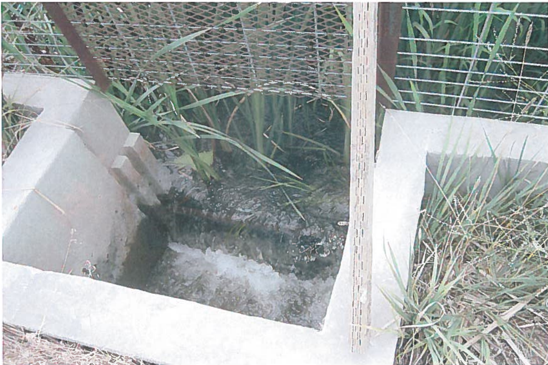
Structure 6, outlet to the slough north of cell # 3.
