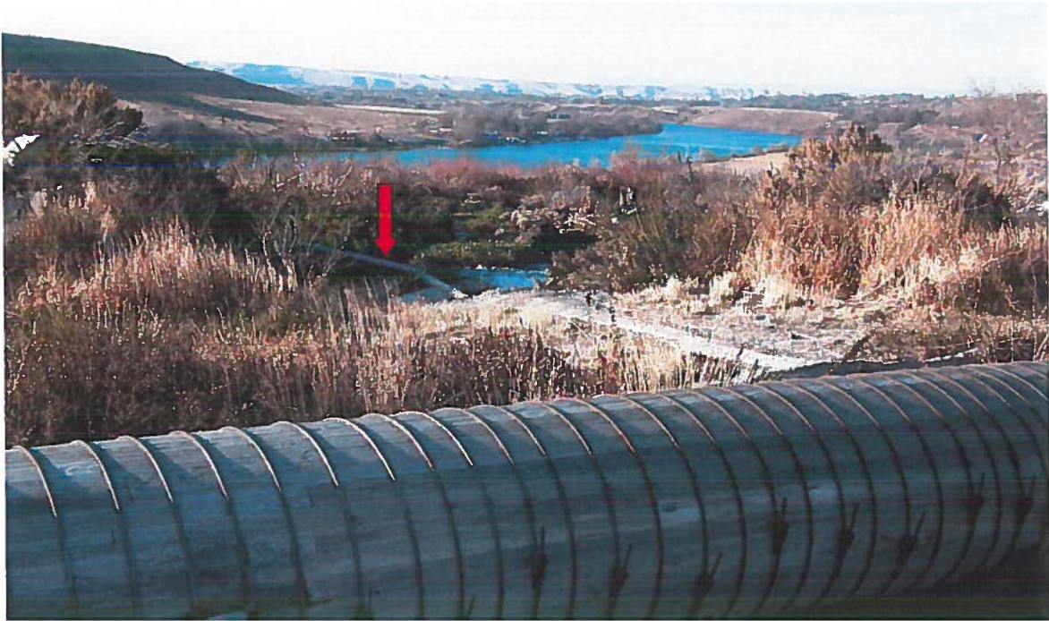
Point of Diversion- Note compressed air pipeline returning to hatchery(Arrow)
