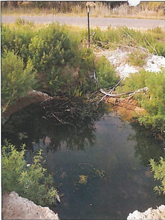
One of the four existing culvert diversions under the highway. Photo looks south across highway to East Side Ditch.
