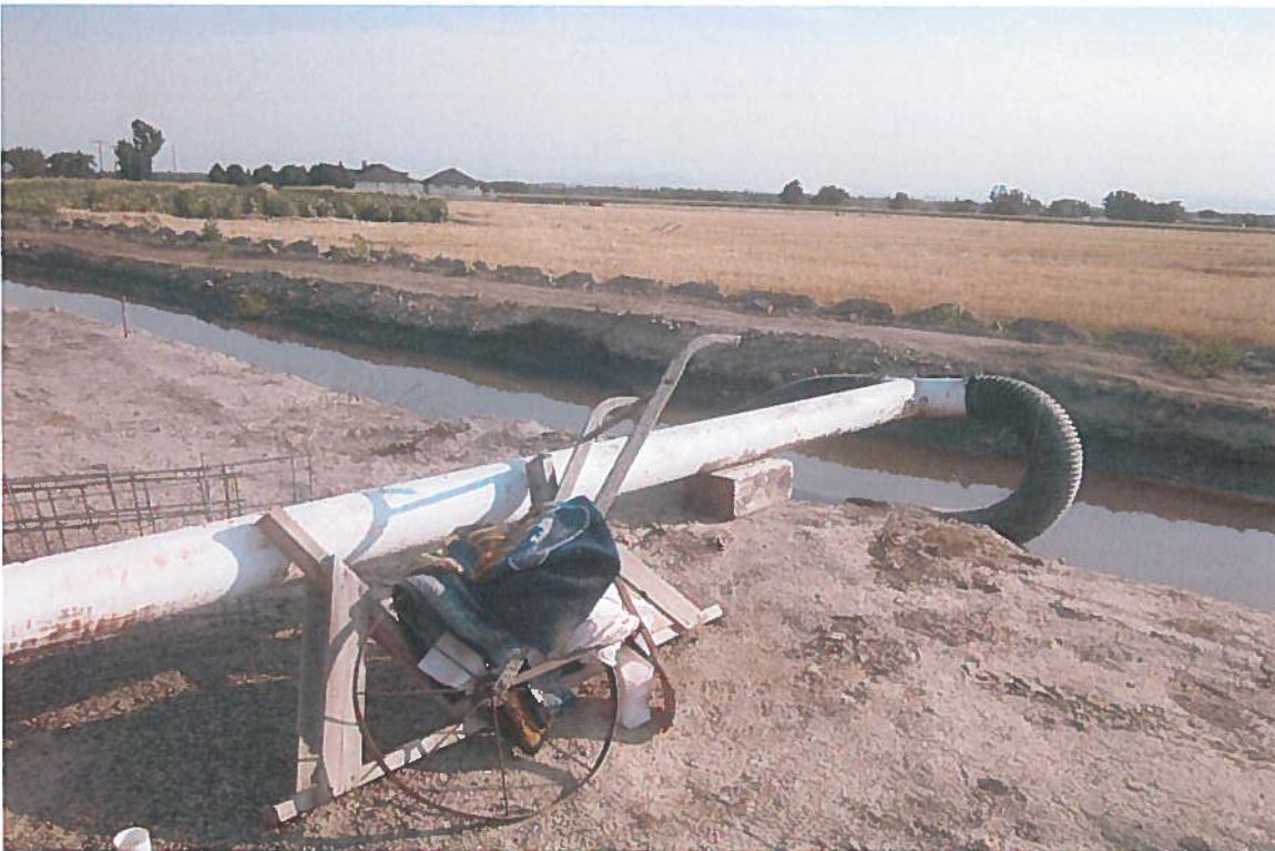
Photo above is the well and motor. White steel pipe seen above and below, which diverts water to a dirt ditch. The dirt ditch is the common surface water and ground water conveyance system.
