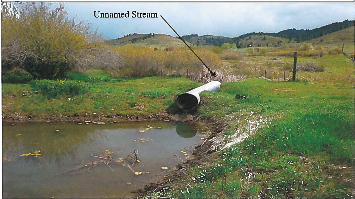
Point of Diversion: View northeasterly of the 36" CMP diverting from an unnamed stream to an irrigation and wildlife storage pond.
