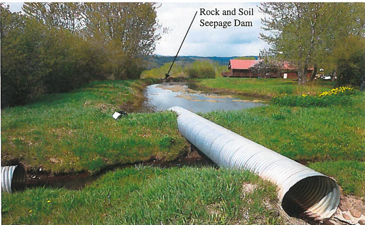
Point of Diversion & Place of Use: View westerly of the 36" CMP discharge pipe and the irrigation and wildlife storage pond. The small ditch beneath the 36" CMP discharge pipe is an irrigation diversion from Grossen Creek. The right holder has no water right or shares from Grossen Creek to beneficially use the water.
