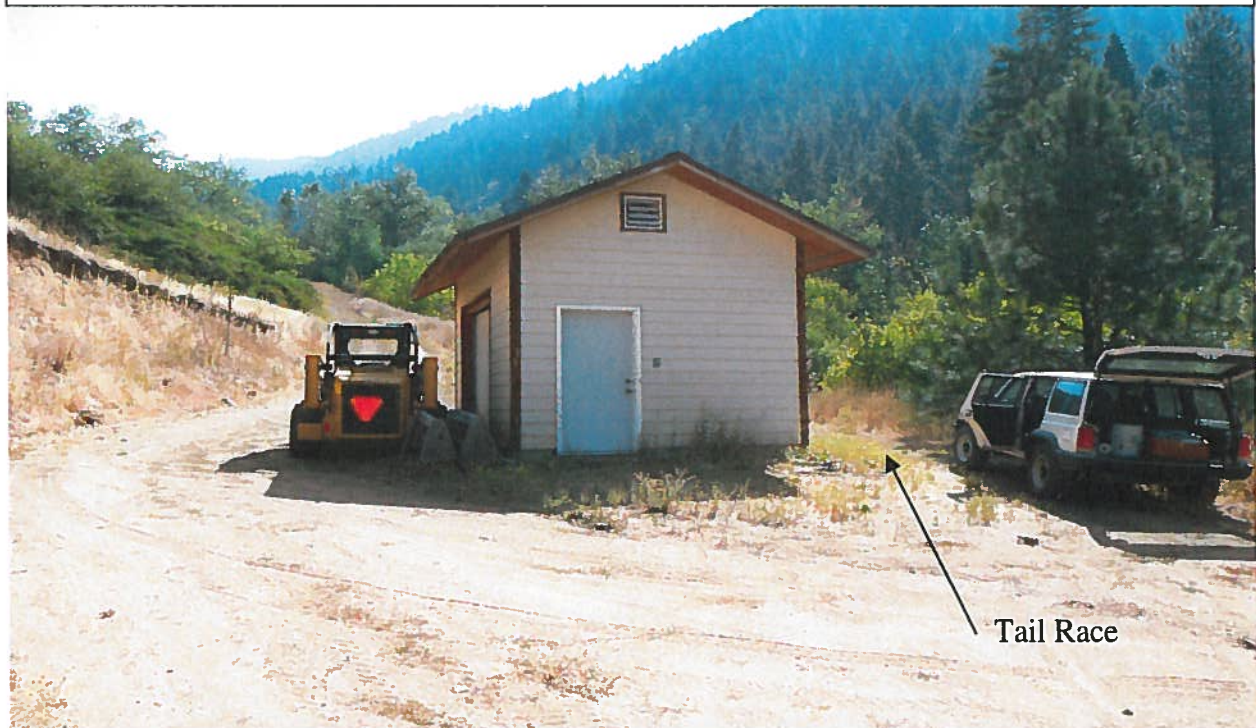
View easterly of power plant. The tail race with discharge back to Hat Creek is located on the south side of the power plant.
