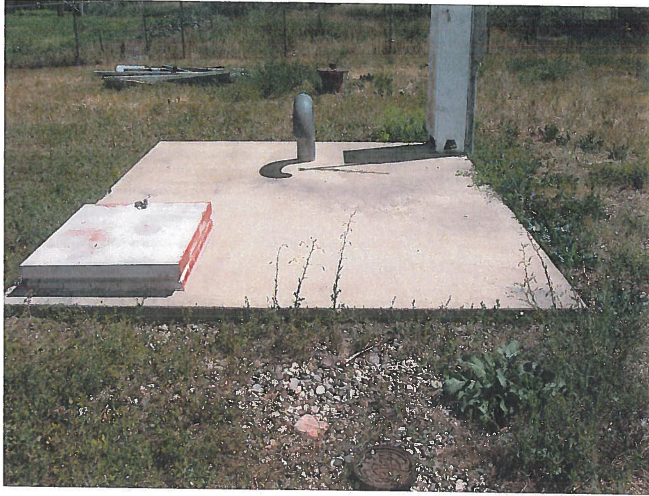
Well #2 Concrete vault
