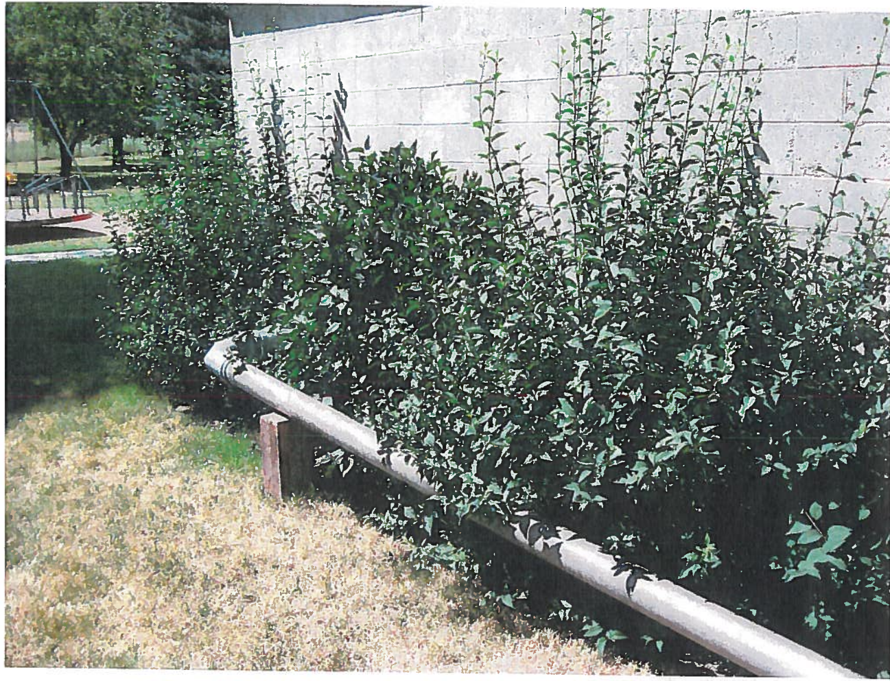
Line running from pump house to park lawn.
