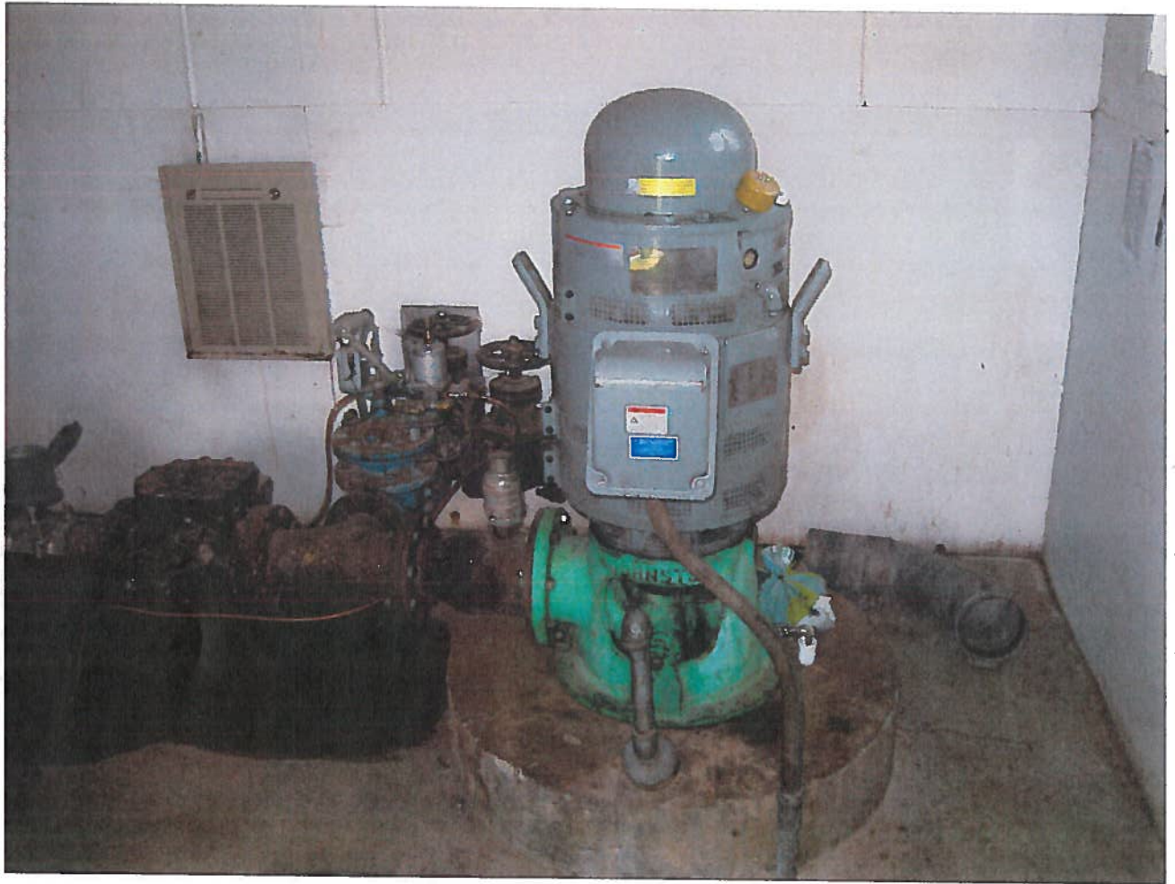
Well #1 40 hp pump
