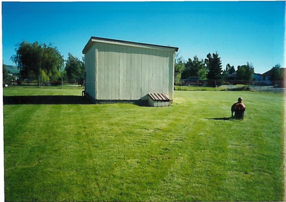
South Park pump house looking South. well in far ground is # E7287 - 20 Hp pump.
