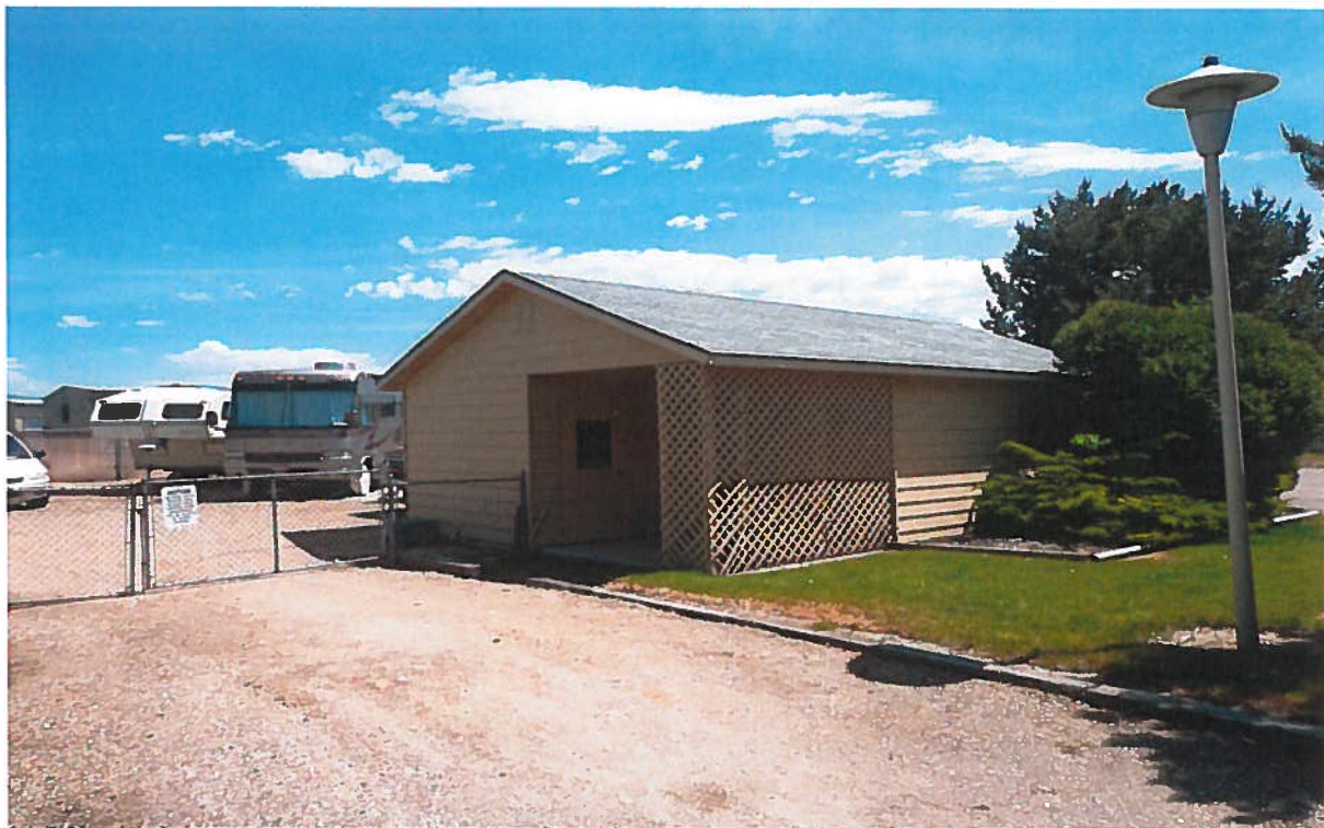
View southeasterly of the pump house located at the southeast corner of the development.
