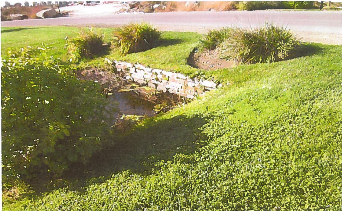
Outlet from pond # 6 to pond # 7.
