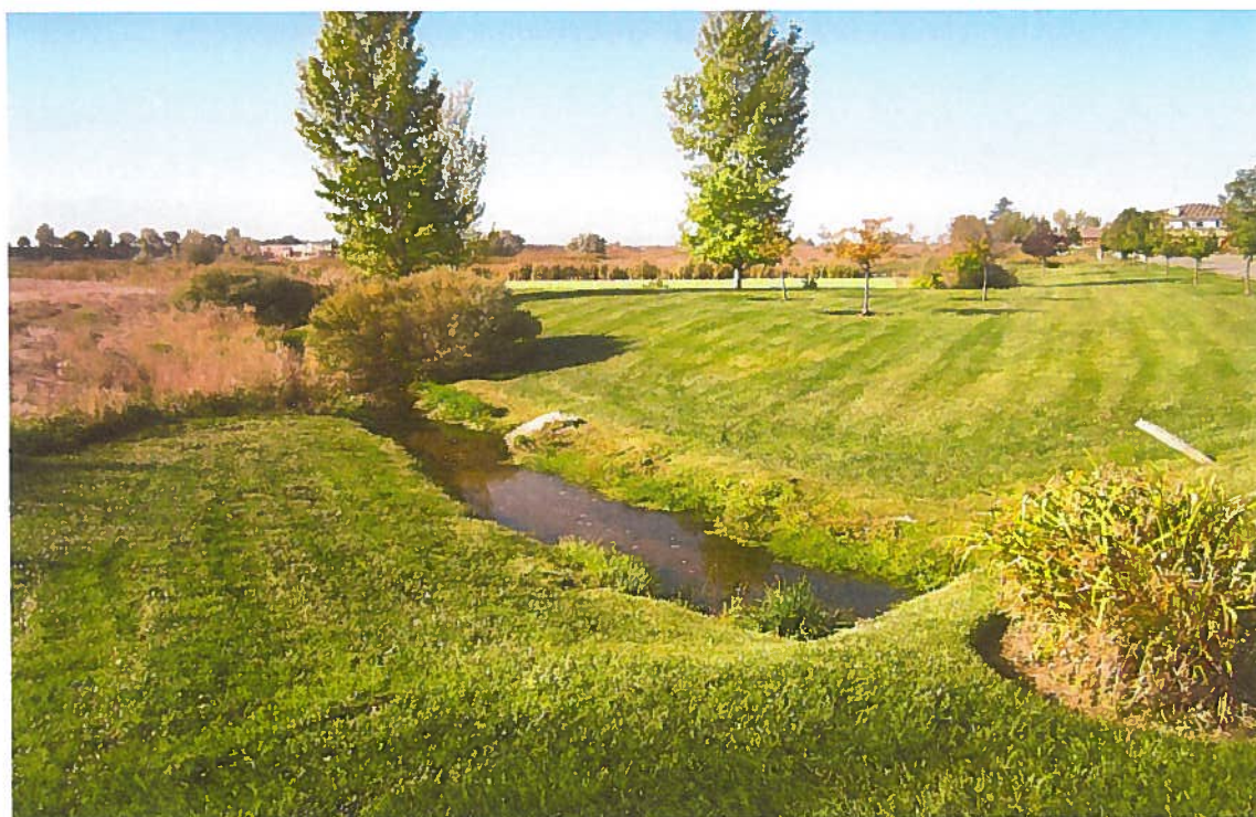
Culvert from pone #4 to pond #5.
