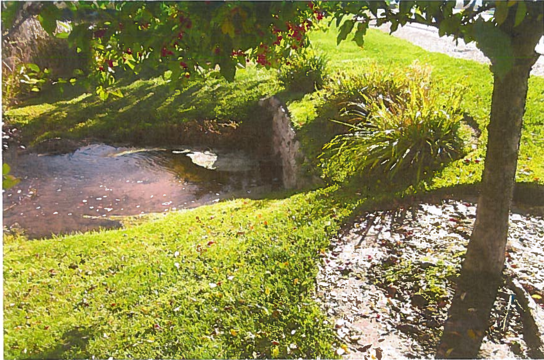
Outlet from pond # 5 to pond # 6.
