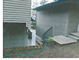
HOME #1 WATER LINE.JPG
