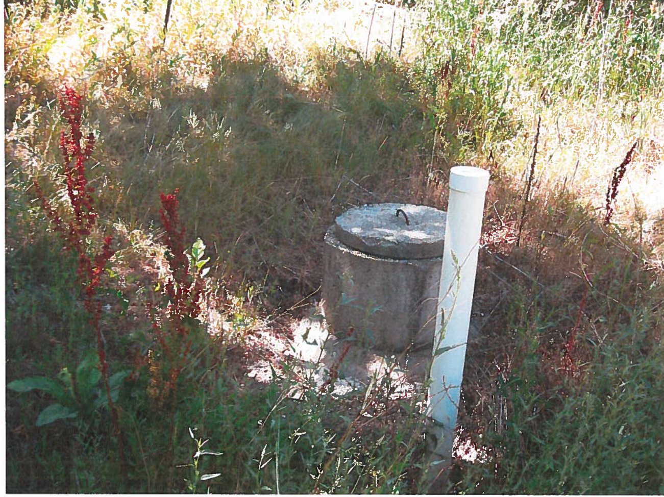
concrete spring box
