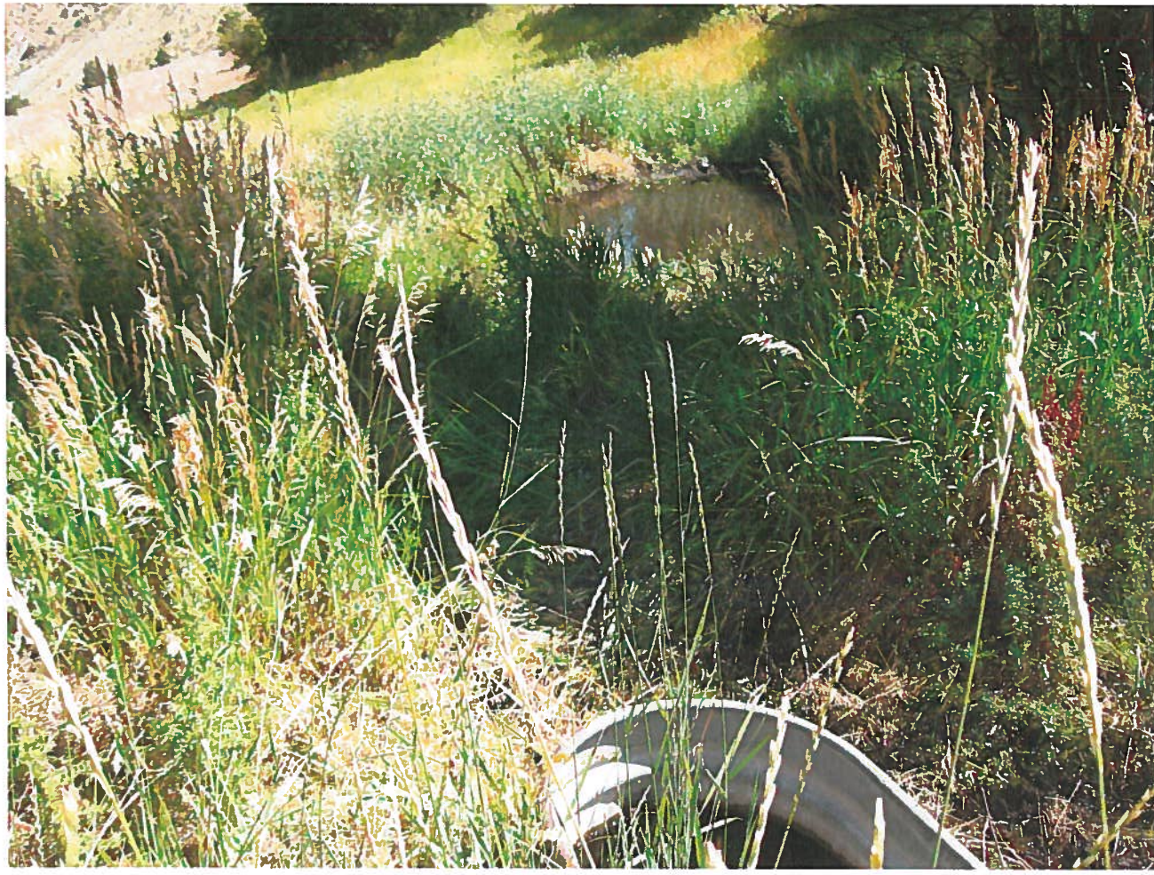
overflow from trough to small dug-out pond
