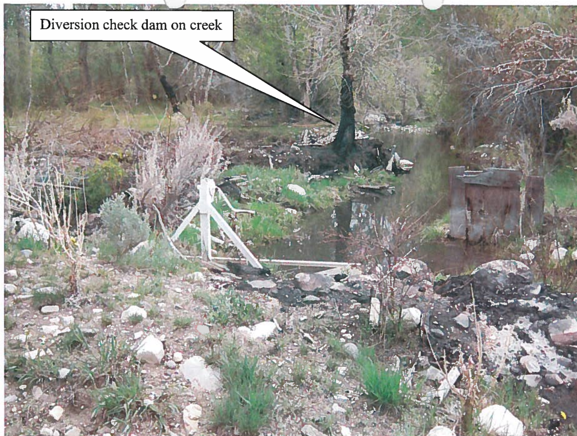
3. Control head gate to Whittaker's Ditch – permit 74-15613.
