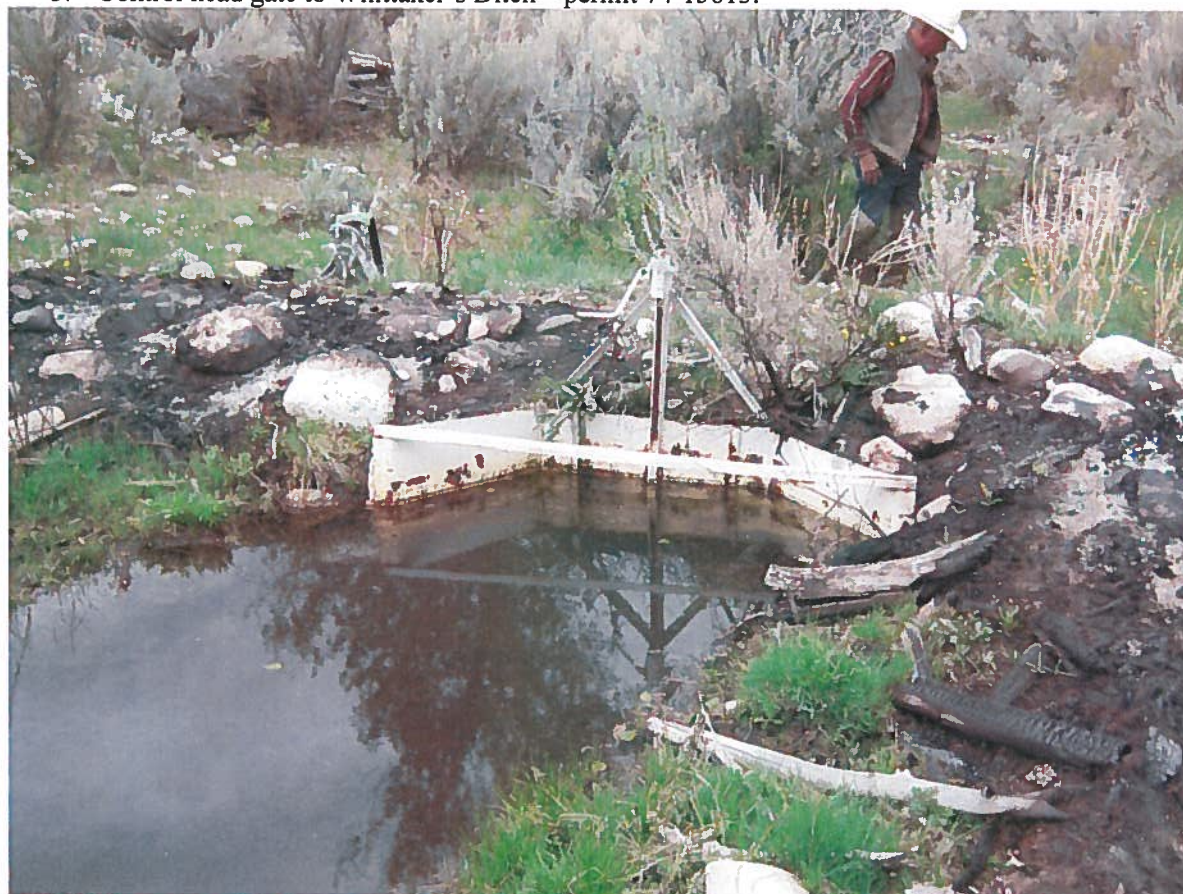
4. Control head gate with ditch in background behind Mr. Whittaker.
