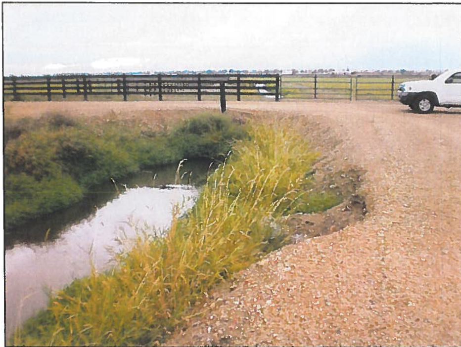
19: Parma Canal facing downstream with flow leaving place of use discharging from culvert pipe.
