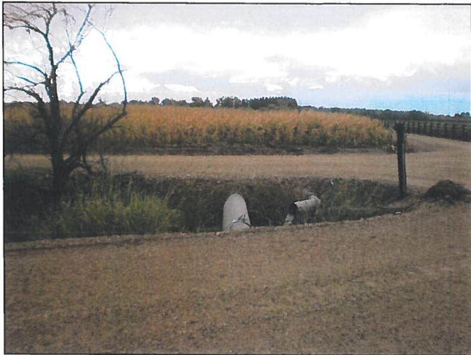
17: Facing west, Sand Hollow Creek water is conveyed via culvert pipe across the drain to the field to west where it flows westerly to the place of use.
