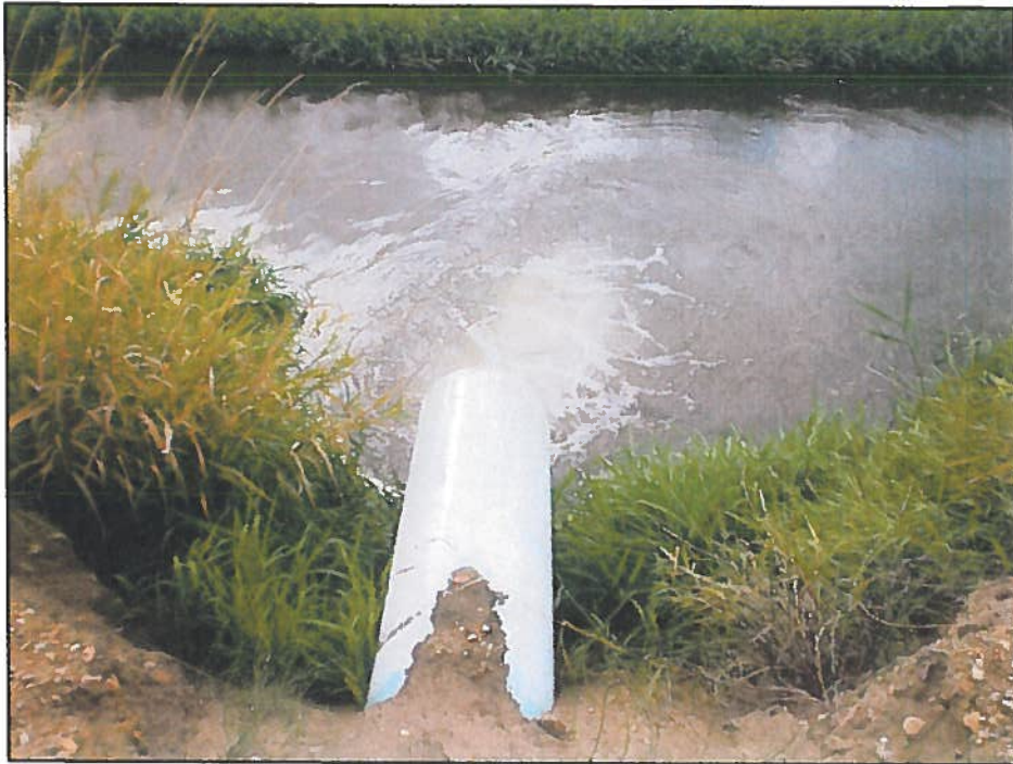
20: Ground water sourcing from pond to the southeast is discharged to Parma Canal.
