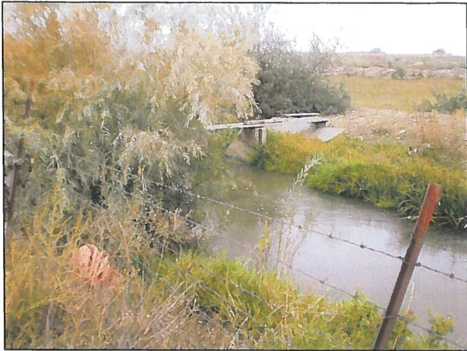
HWY 95: Check structure in Sand Hollow Creek at Highway 95. Headgate under branches to photo left.
