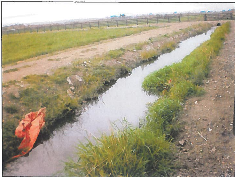
18: Lower takeout from ditch are two 11-inch pipes on photo right at orange tarp.
