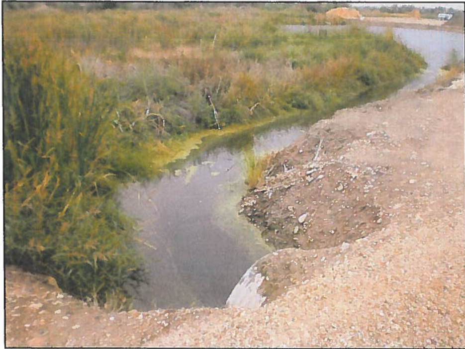
19: Water leaving place of use and entering culvert pipe to flow into Parma Canal.
