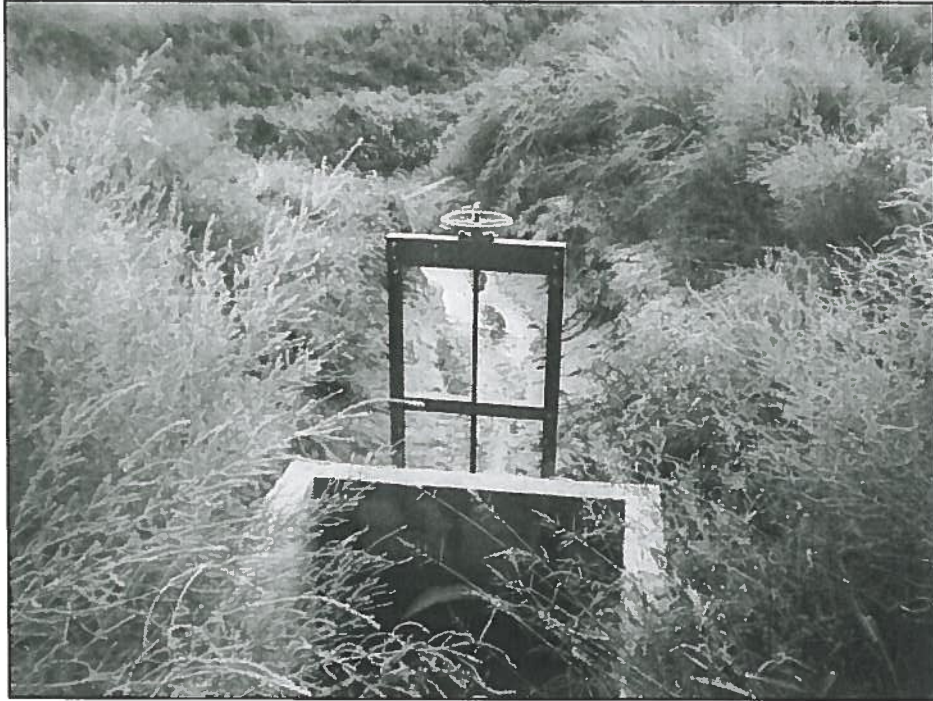
23: Upper Haas Ditch diversion headgate from Baldrige-Meadows Drain.
