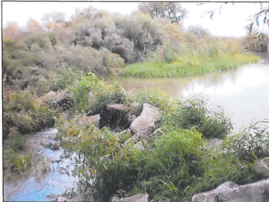
21: Rubble check structure. Photo taken on left bank of left side channel facing across check structure to McConnell Island.
