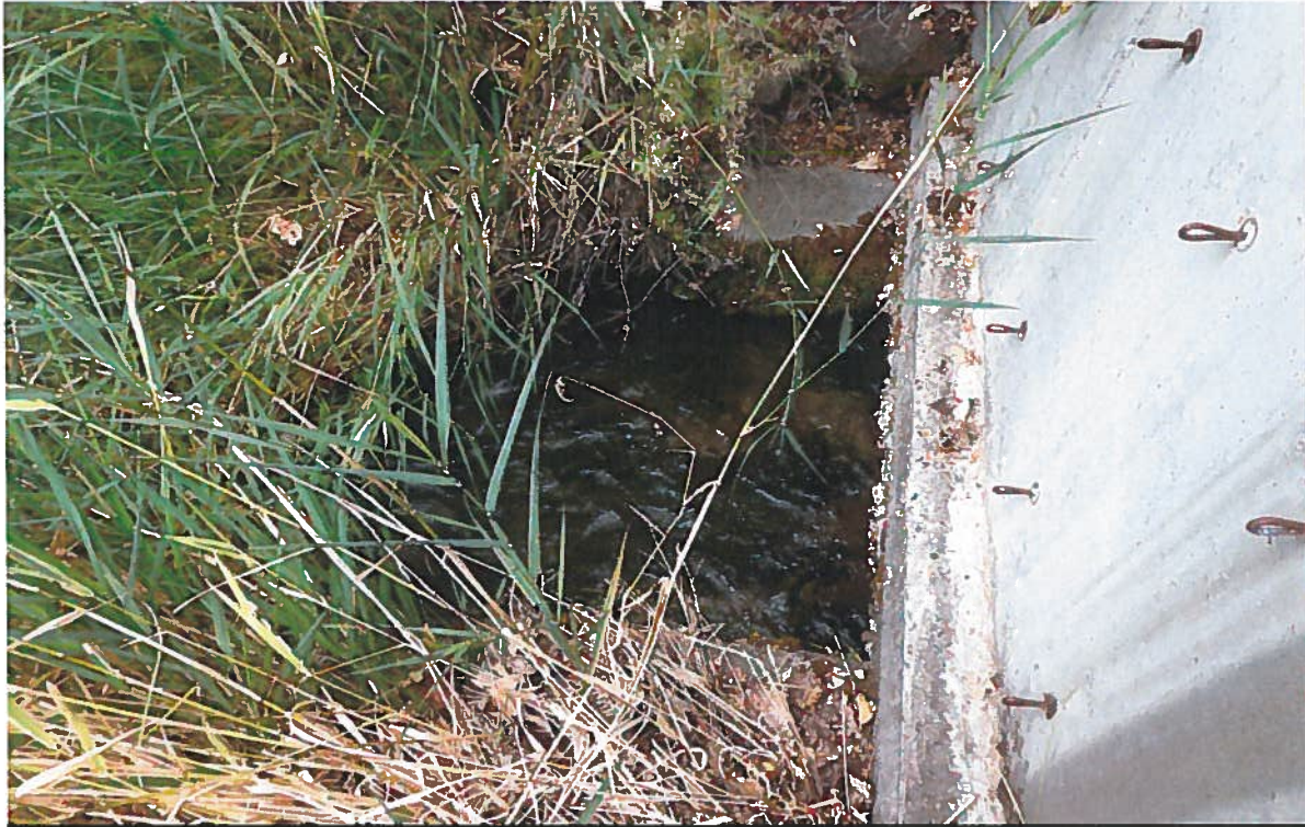
View of raceway channel discharging back to the West Fork of Race Creek. Since the date of this photo, the right holder has installed a rectangular weir for flow measurements in the raceway.
