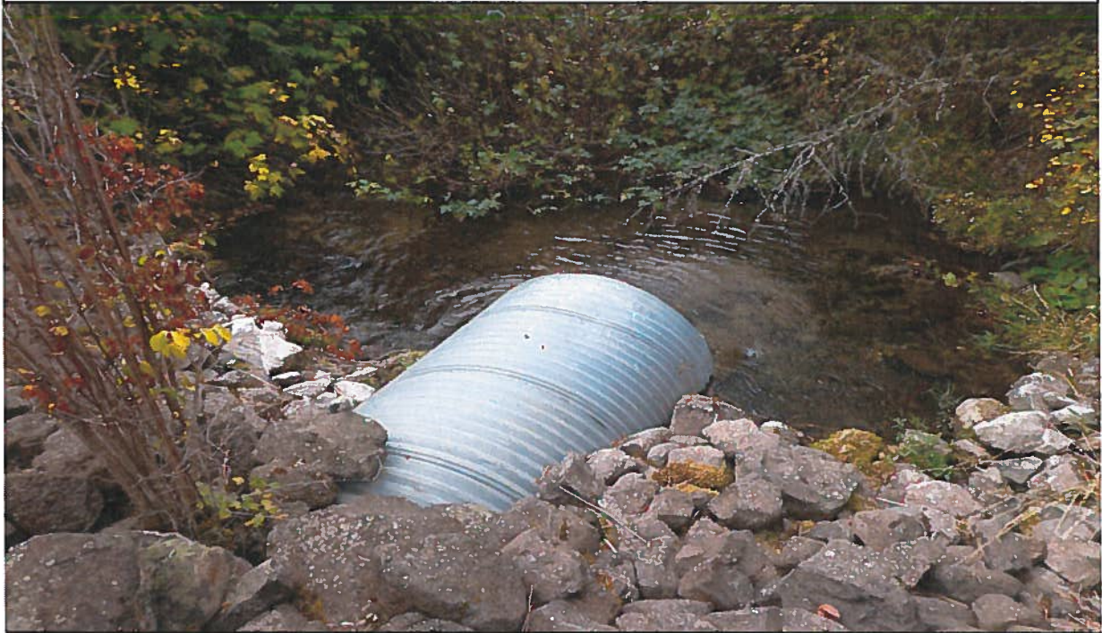
Point of Diversion: View westerly of the 48" diameter CMP culvert which diverts water from the West Fork of Race Creek to a concrete diversion structure.
