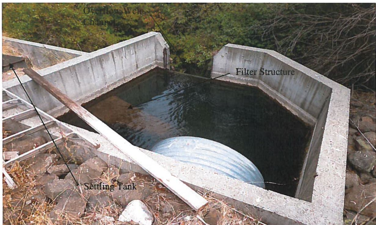
View easterly of the 48" diameter CMP culvert discharging to the concrete diversion structure. The overflow weir channel discharges water back to the West Fork of Race Creek. The submerged structure is a filter for a 4'x4' concrete channel which discharges water to a settling tank.
