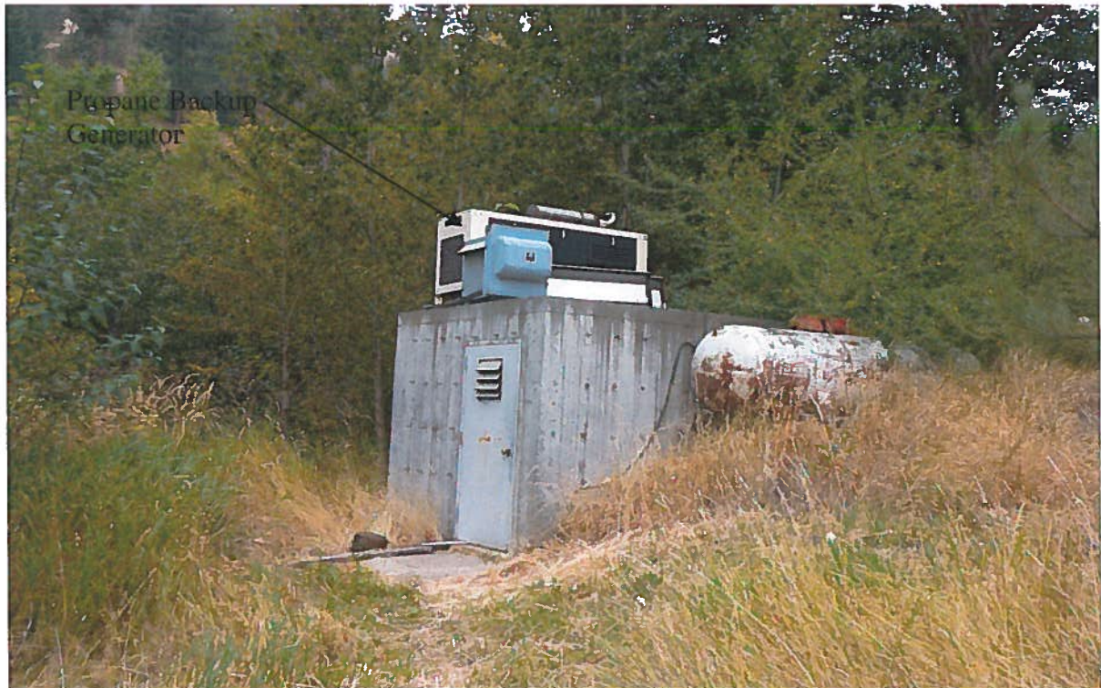
View westerly of the power house located north of the West Fork of Race Creek.
