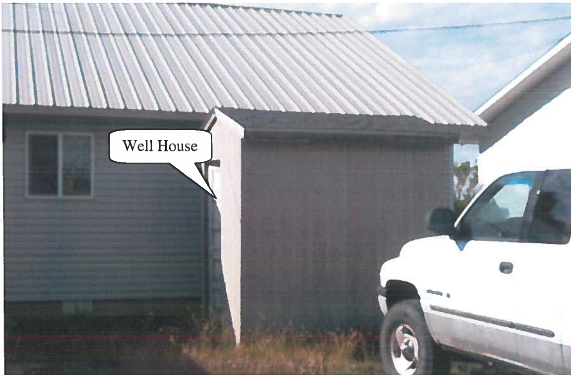
Backyard of Residence looking South
