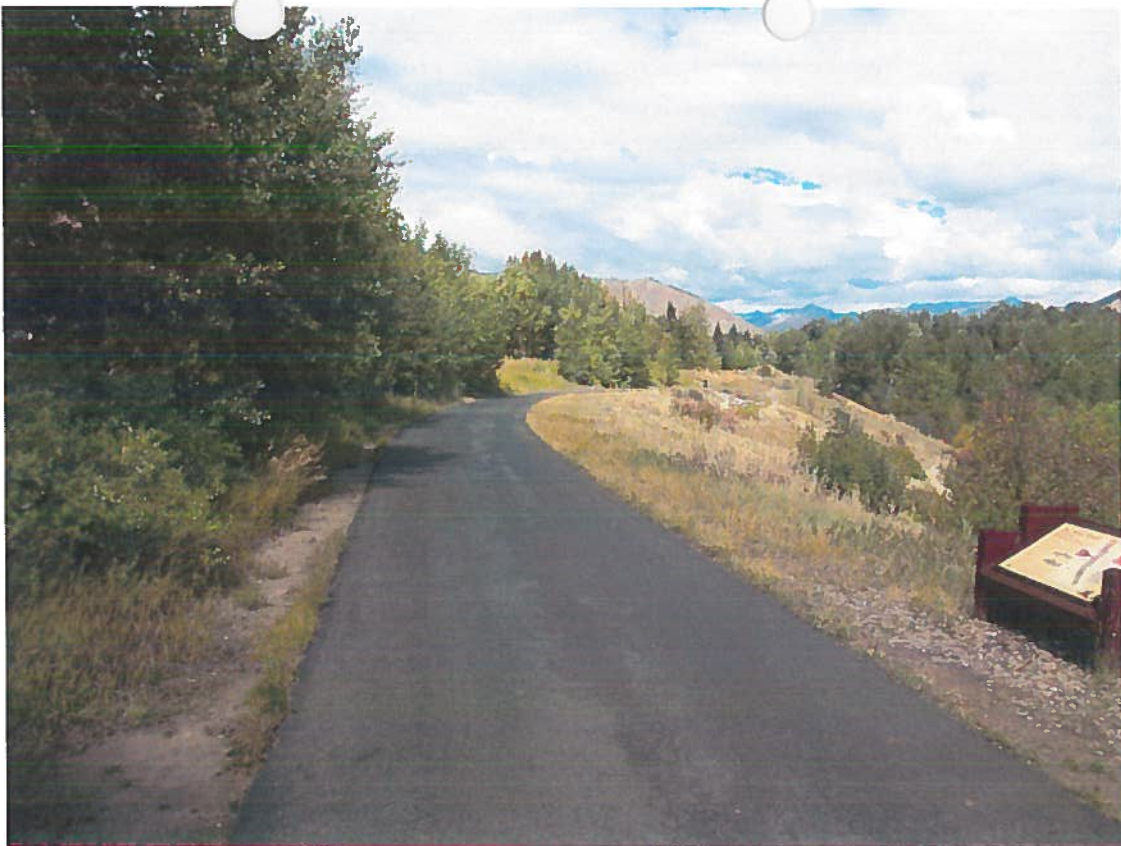
Middle portion of the project, looking north
