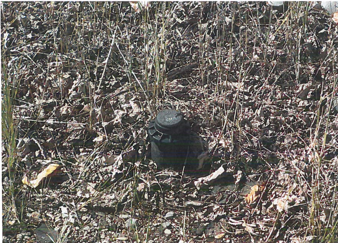
Sprinkler head along pathway
