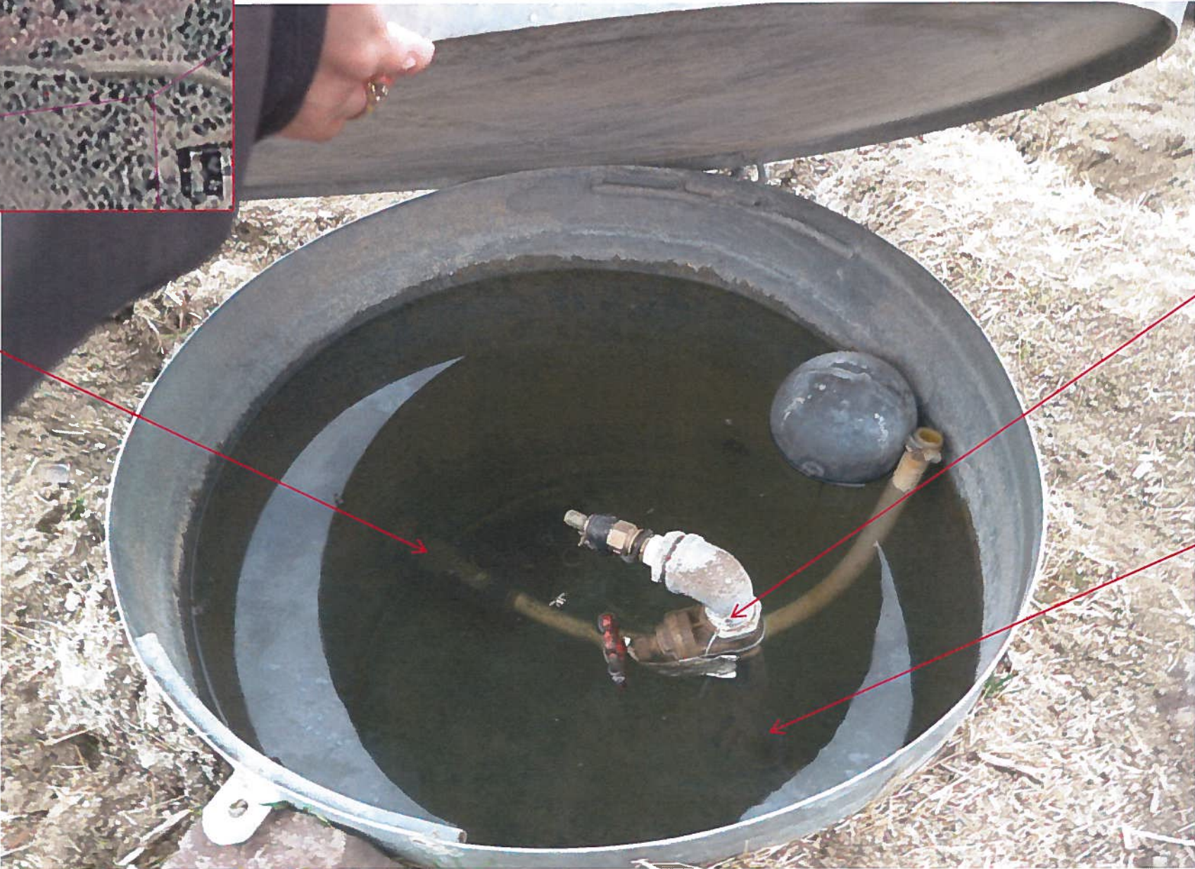
Picture of shutoff valve inside of valve can.
