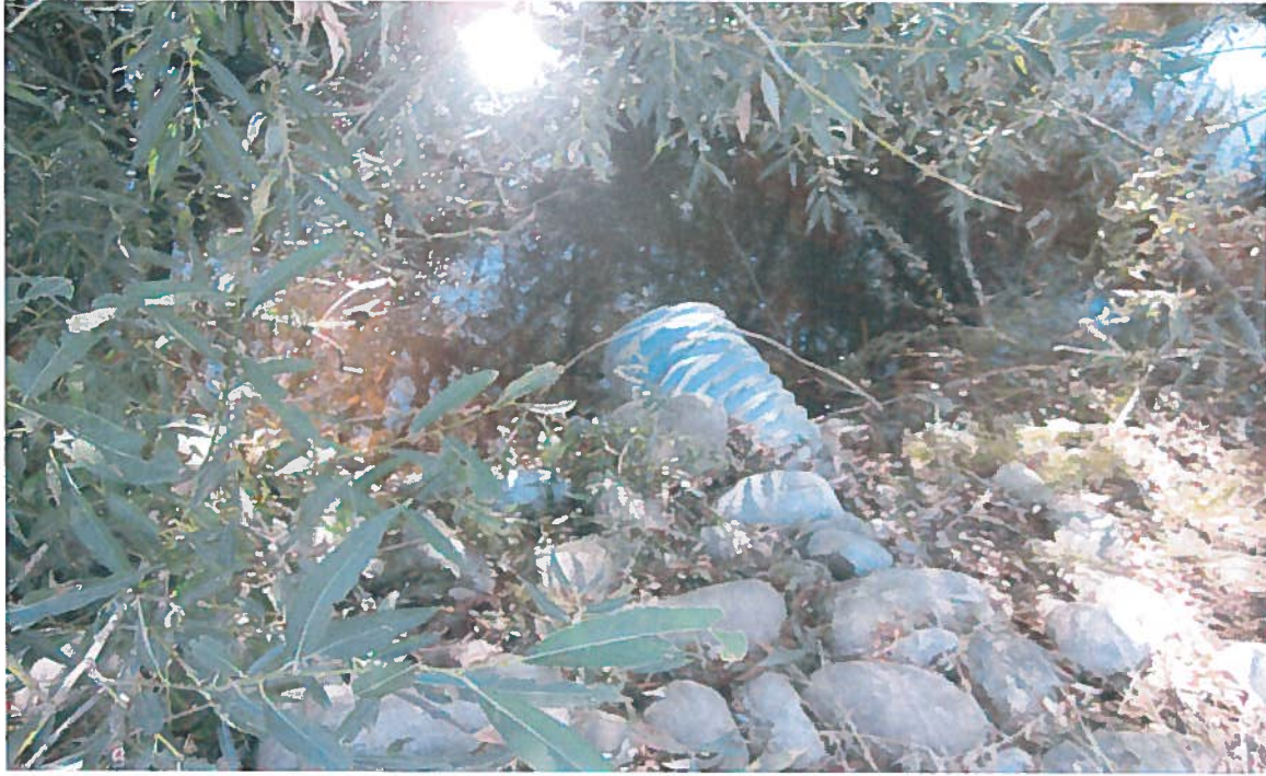
Outflow pipe to Middleton Mill ditch.
