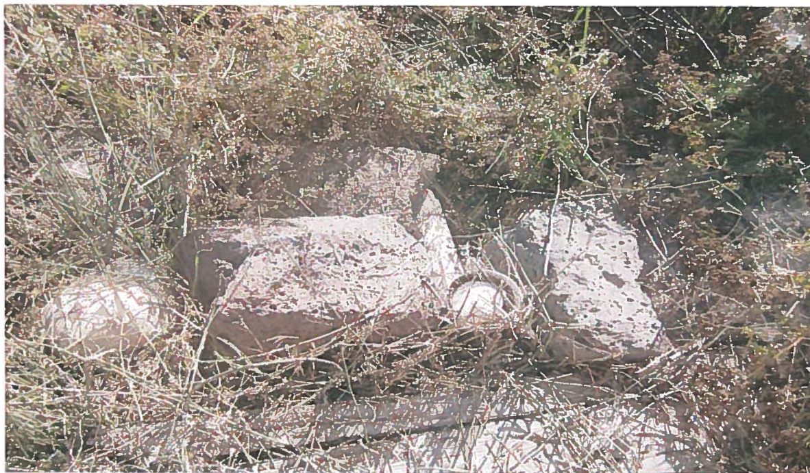
Inflow pipe to pond for water that drains from the nursery.
