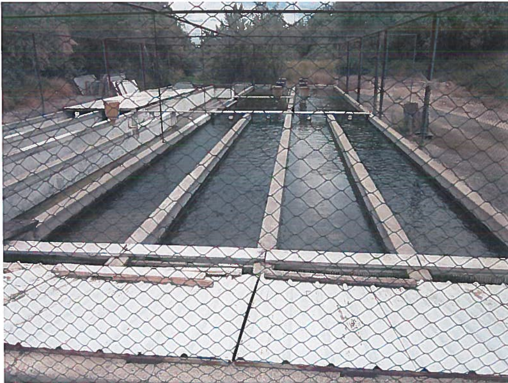
Figure 4: Raceways from upper end looking northeast
