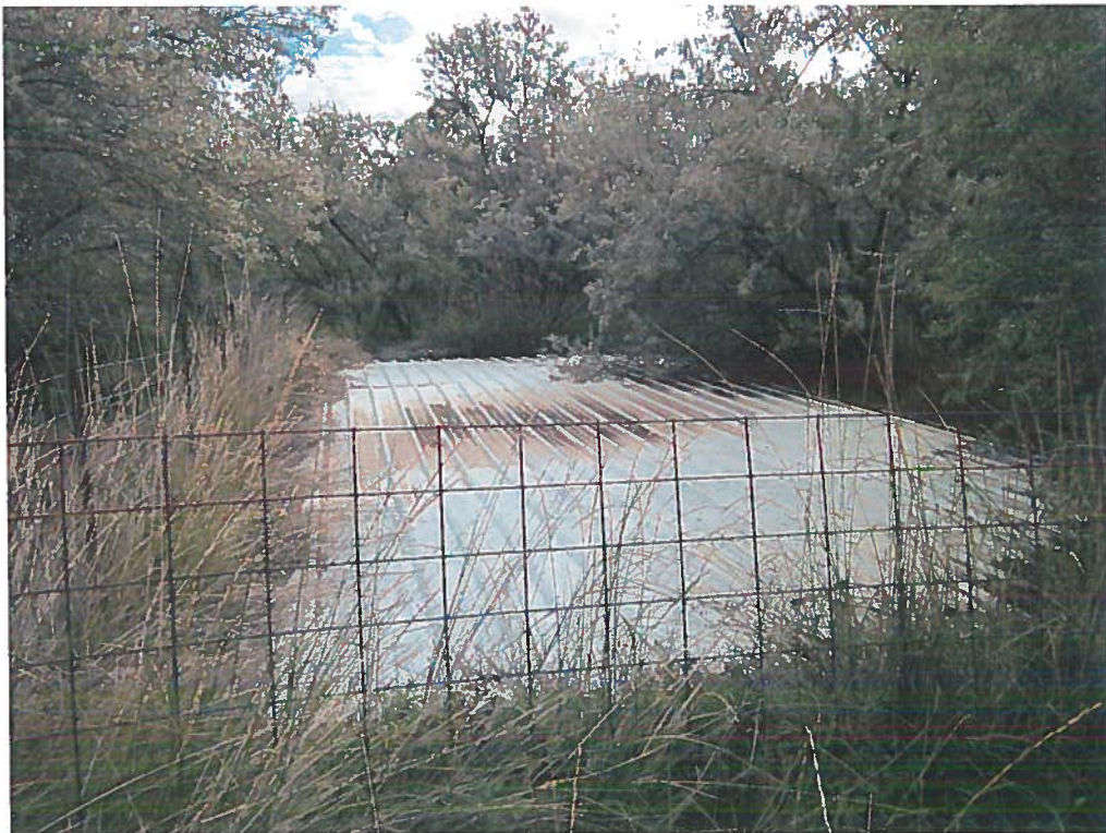
Figure 1: Upper end of impoundment at the point of diversion
