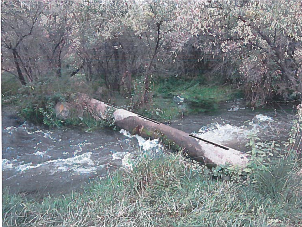
Figure 2: Pipeline crossing Mud Creek
