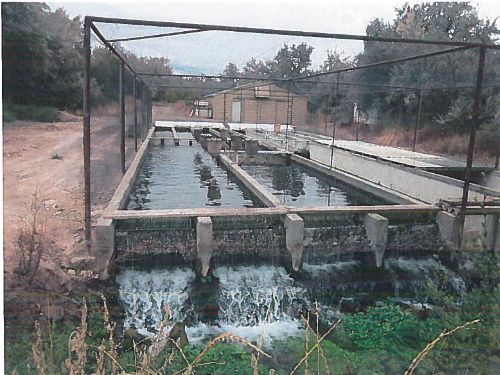
Figure 5: Raceways and hatch house from outlet looking southwest
