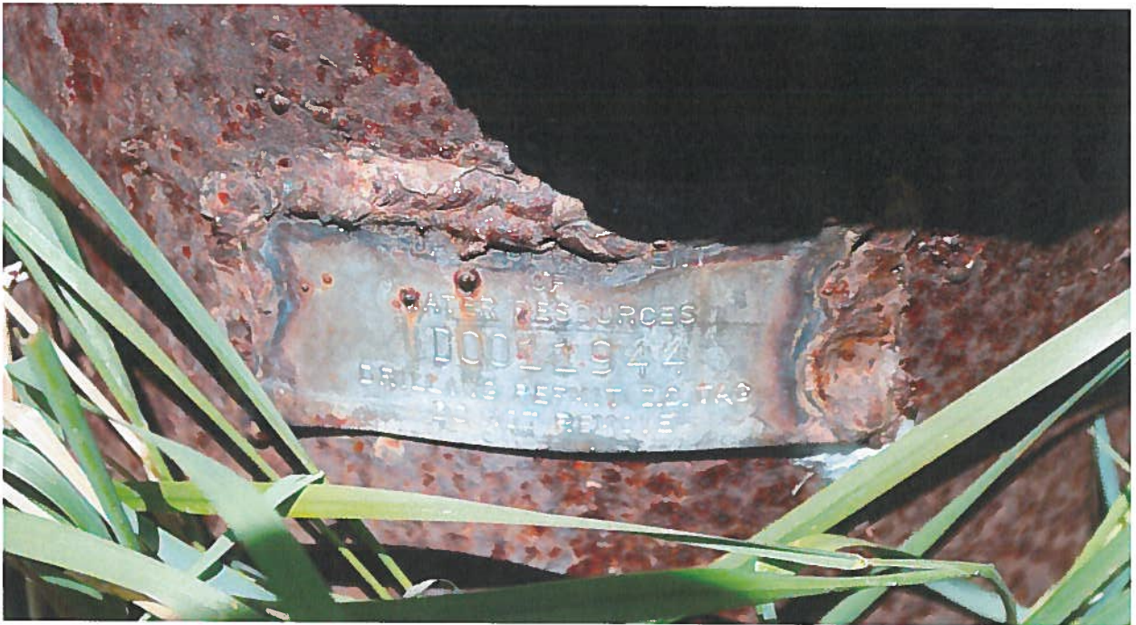
Field Inspection 15-7515 – August 28, 2012
