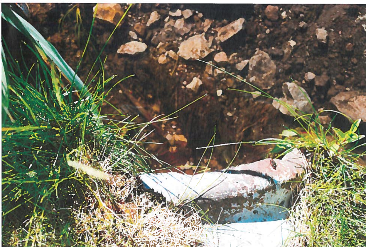
Pond Outlet no screen
