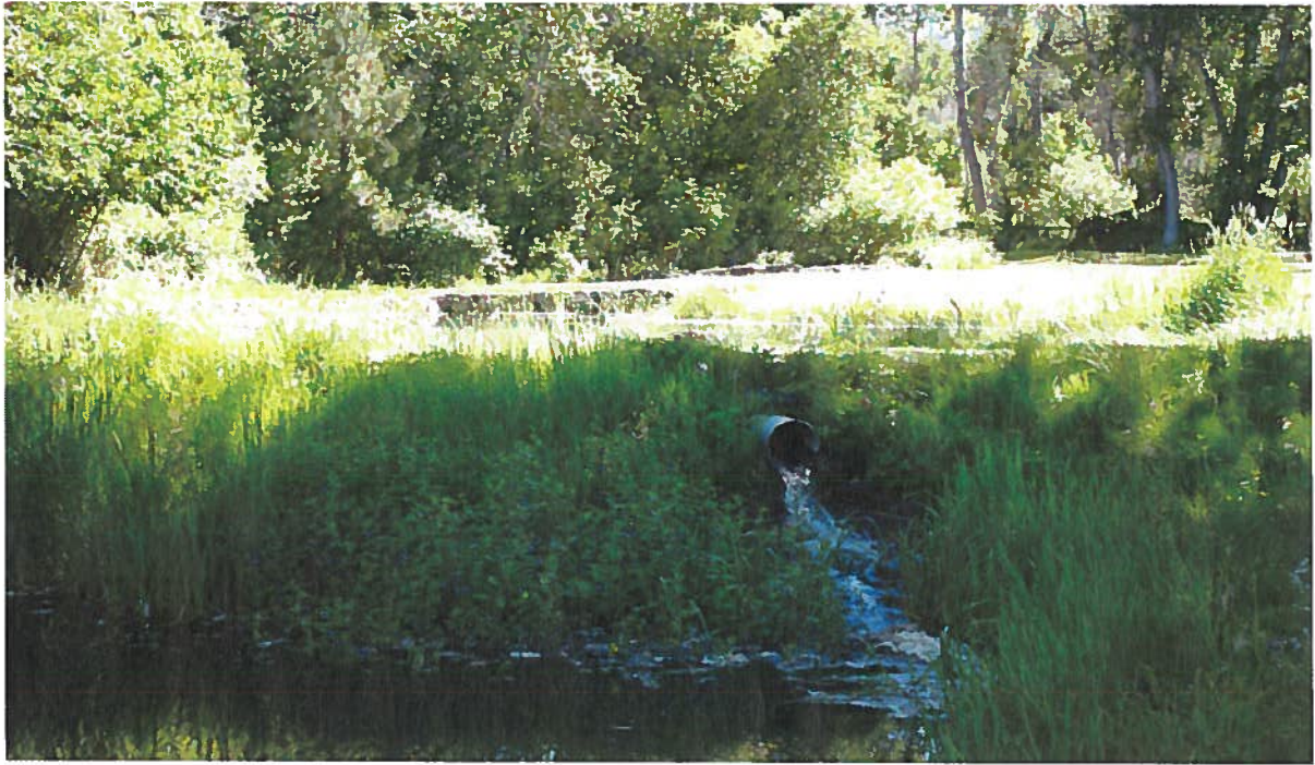
Culvert between ponds
