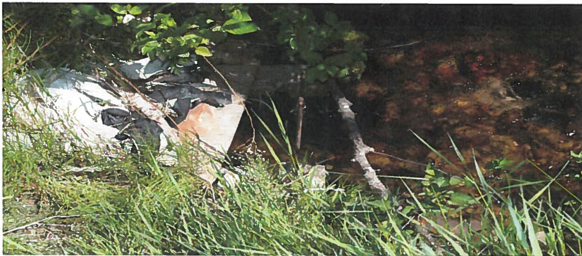
Diversion to Ponds off of Tower, no fish screen
