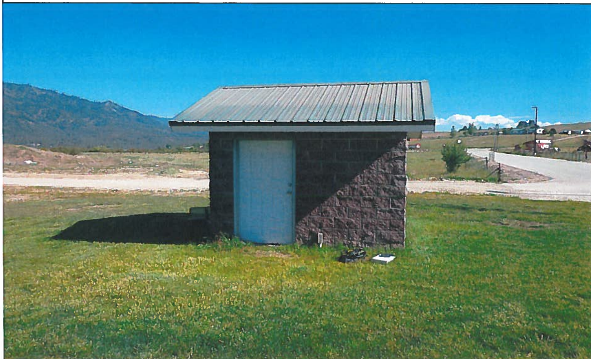
Point of Diversion: View northwesterly of the well/pump house.
