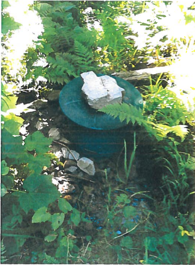
Spring Box at Point of Diversion
