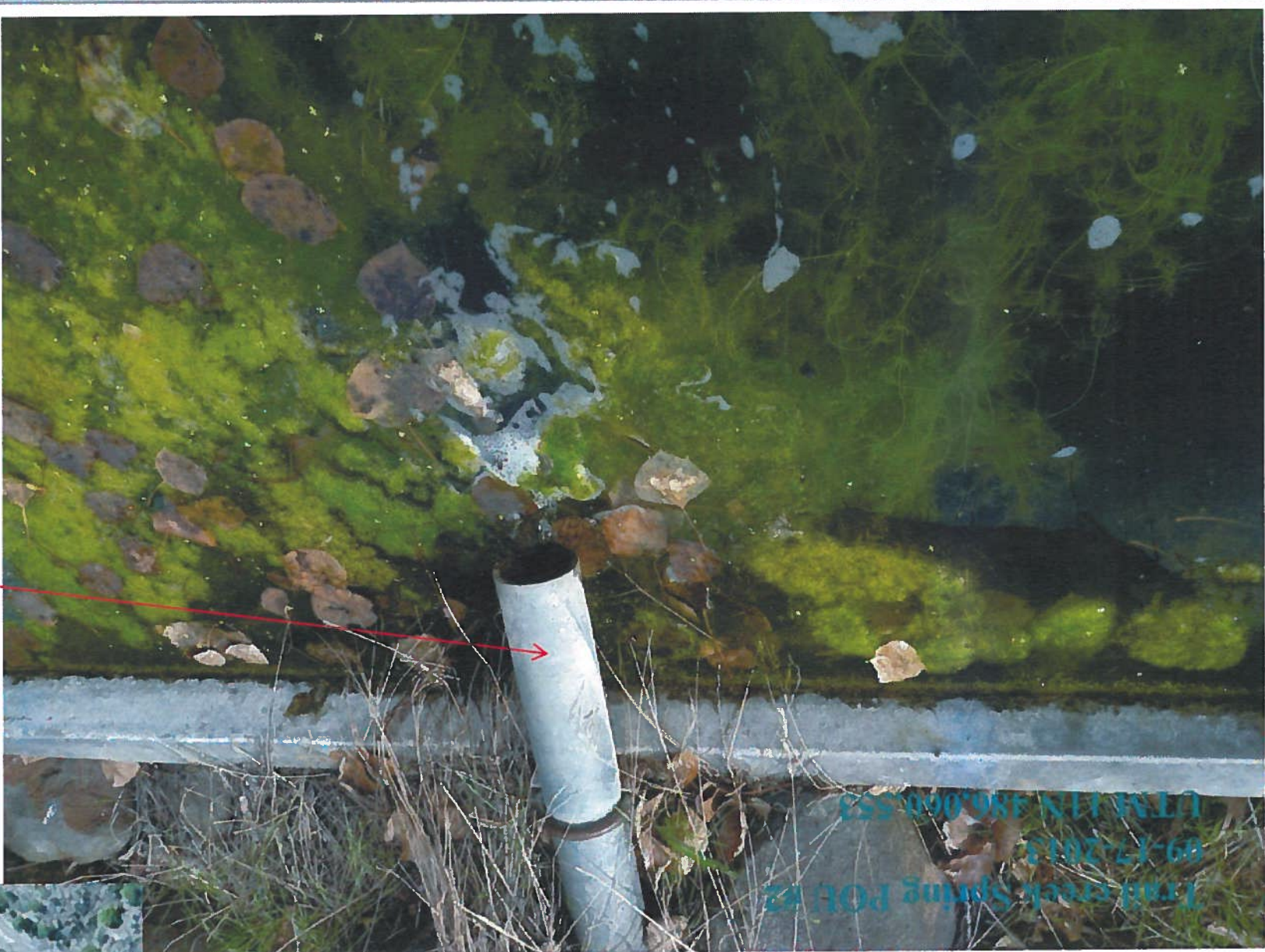
Picture of Inlet of trough #2
