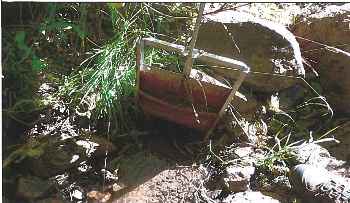
Point of Diversion: View westerly of a 10" slide gate at the head of an excavated ditch. Approximately 10 – 12 feet of buried 10" CMP culvert pipe diverts water from the Unnamed Stream to the excavated ditch and 10" slide gate.
