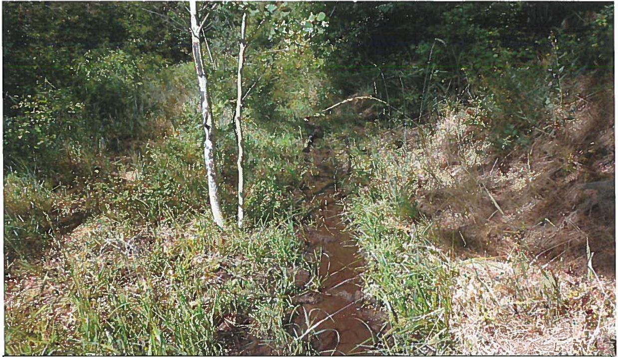
View westerly and upstream of the excavated ditch which conveys water to a pond known as the 'Cabin Pond'.
