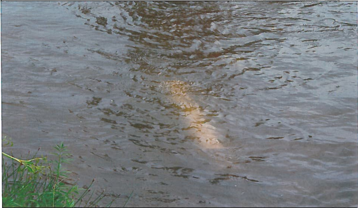
Point of Diversion: View easterly of the submersible pump 4" PVC sleeve near the west bank of the Middle Fork of the Payette River.
