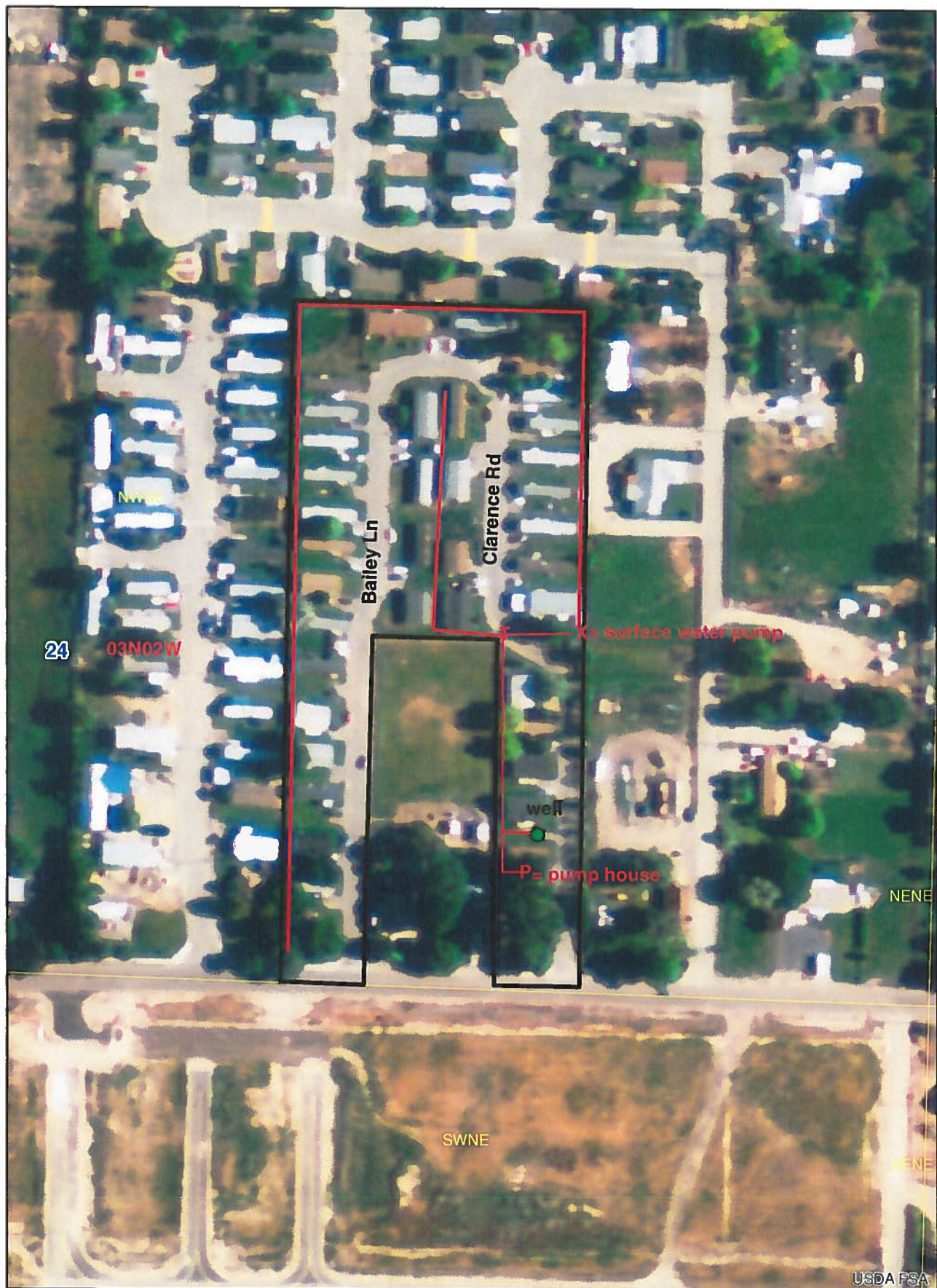
63-12518 - 2011 Bing Photography. Bailey Park. Place of use outlined in black. Ground water and surface water is conveyed through a 3" diameter PVC pipe, shown in red.
