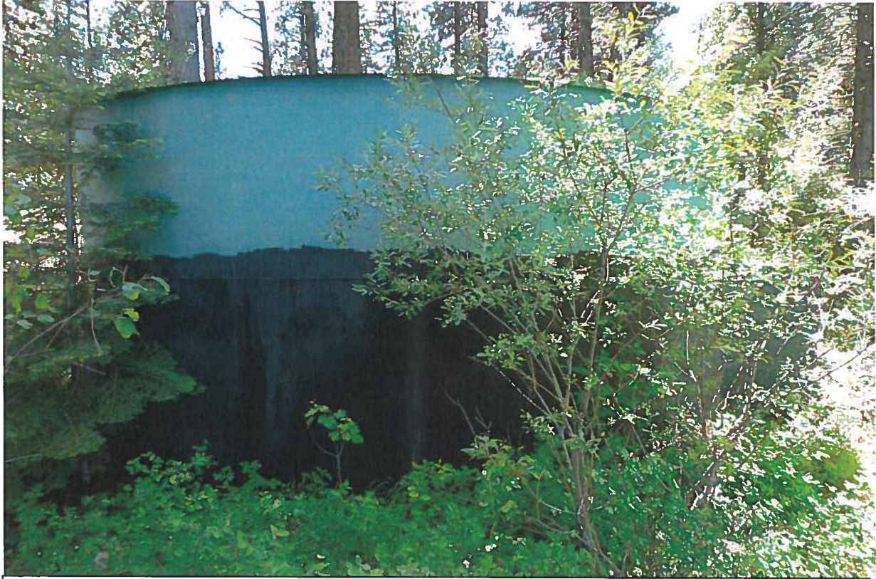
View northerly of a steel 30,000 gallon water storage tank serving the Shiloh Ranch Estates development.
