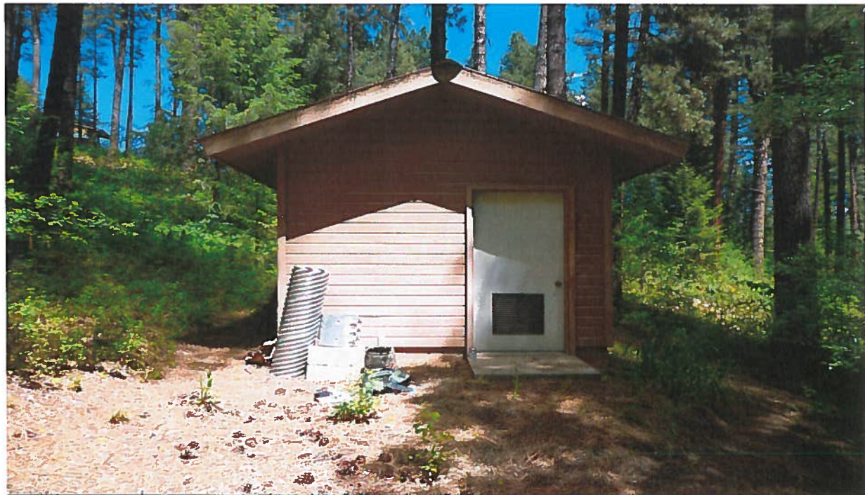
View northerly of the well/pump house located on Lot 27, Shiloh Ranch Estates.
