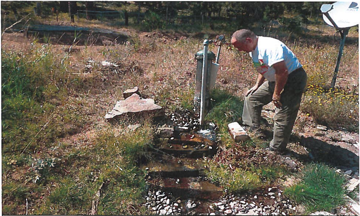
Point of Diversion: View westerly of the artesian well. The well discharges to the east in a drain ditch which discharges into an irrigation/aesthetic storage pond.
