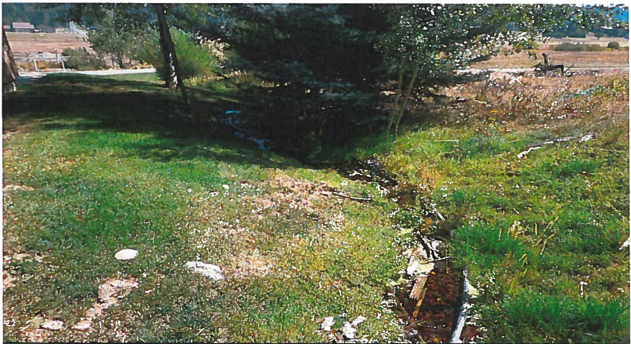
View easterly from the artesian well of the drain ditch which discharges to an irrigation/aesthetic storage pond.
