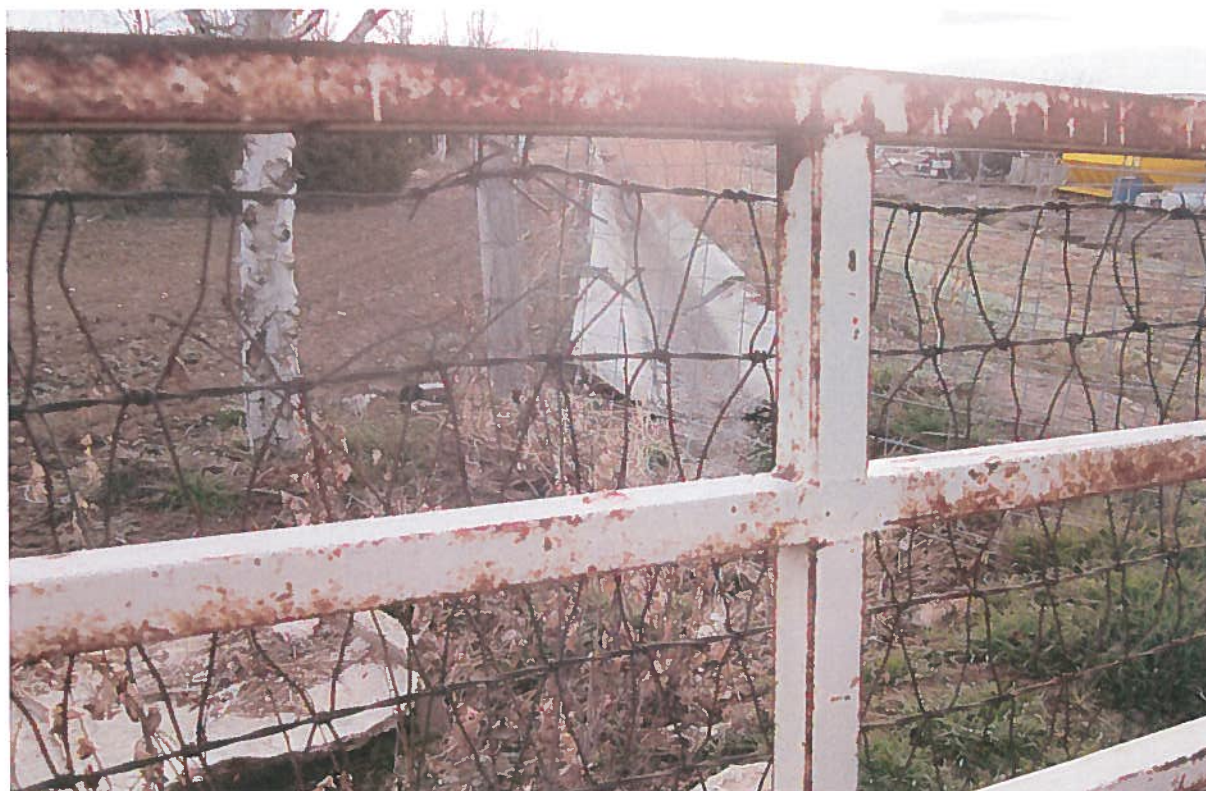
Primary irrigation provided from this NMID ditch through buried pipe.
