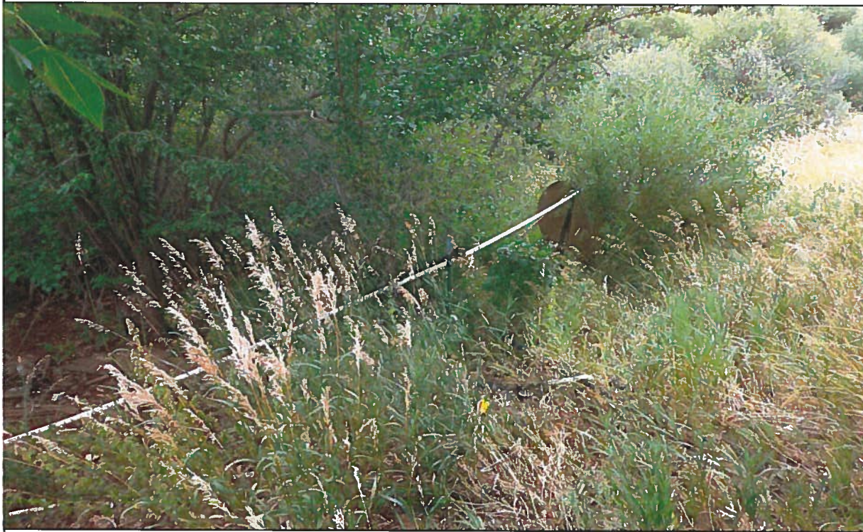
View southwesterly of the 1" PVC supply line from the spring box and a 300-gallon steel water storage tank located southerly of the home.
