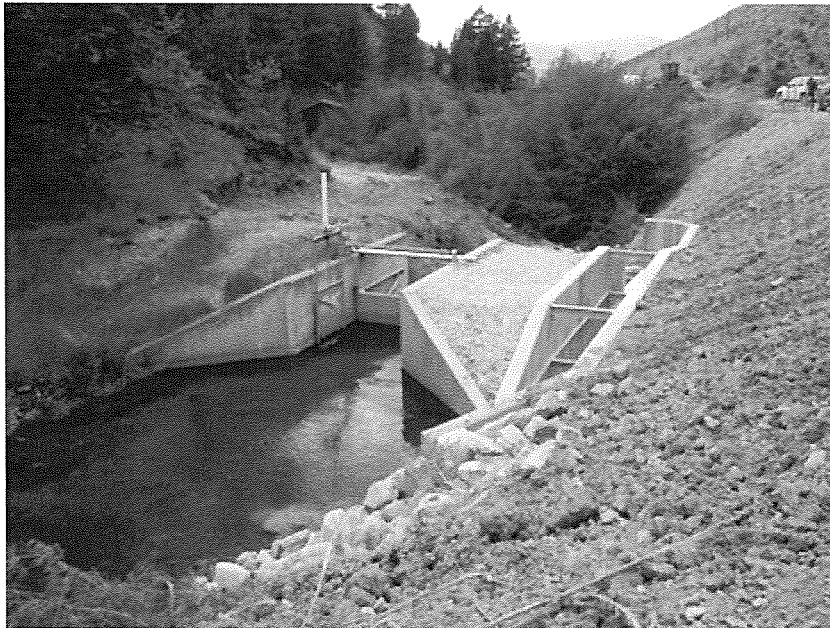
Backfilled fish ladder structure.
