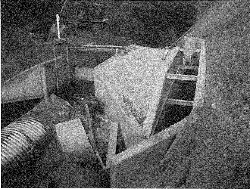
Water diversion into hydroelectric diversion intake so construction crews can work in the dry.
