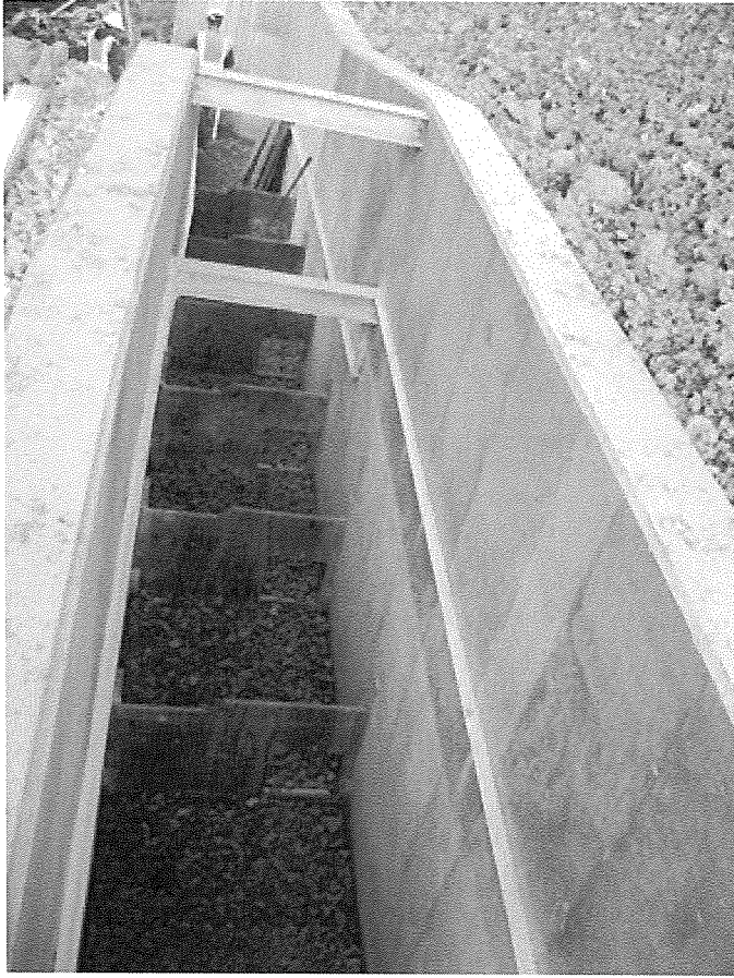
Simulated stream bottom in fish ladder.
