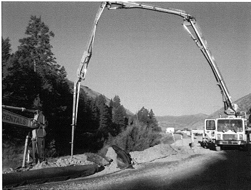
Concrete pumper pouring the floor of the fish ladder facility around the Georgetown hydroelectric diversion headgate, July 2009.
