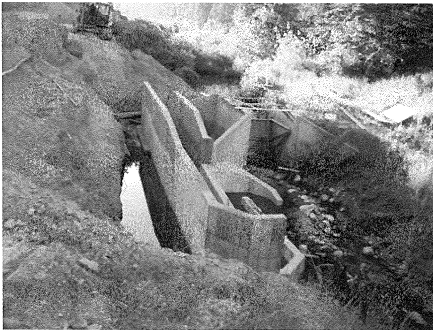
Georgetown fish ladder under construction, July 2009.
