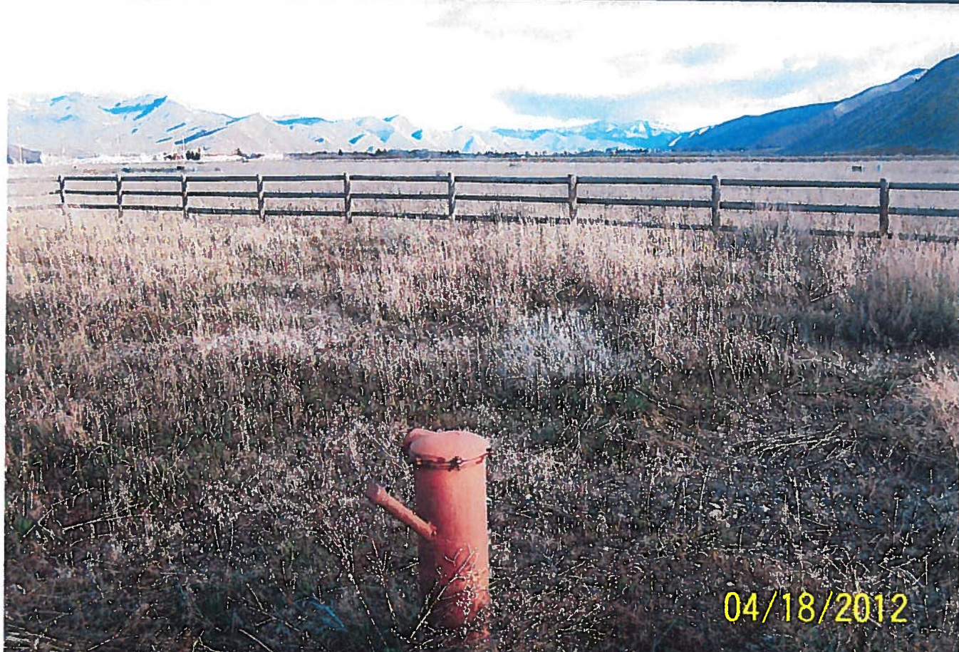
POD North Well D002366 2 1/2" casing 29" above ground level
