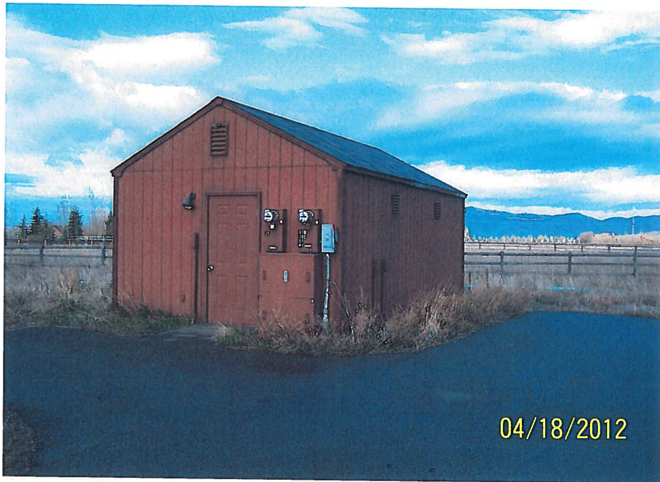
Pump House located on Parcel F Lot
