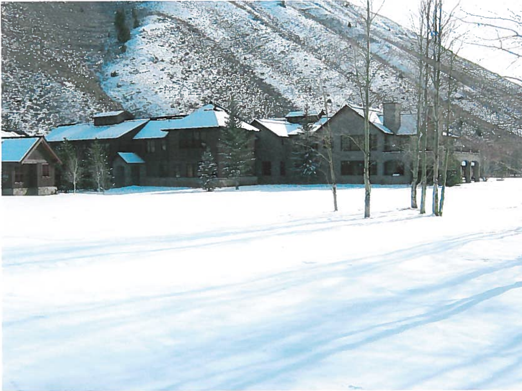
Residence looking southeast
