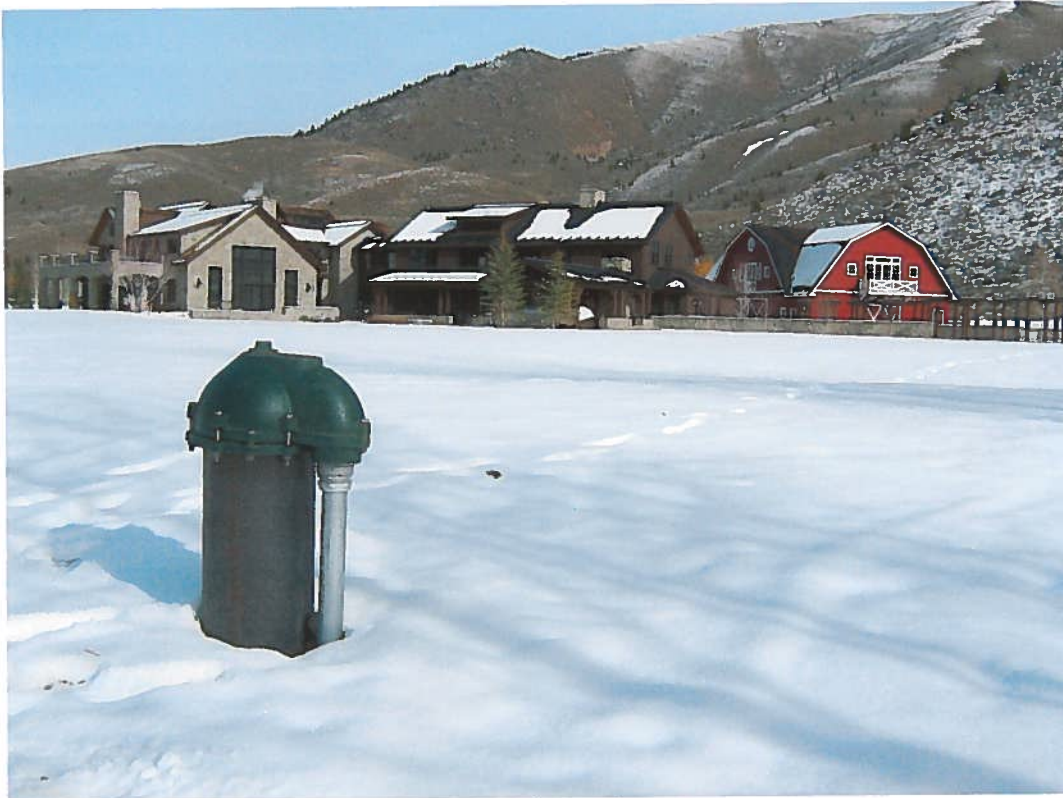
Withdrawal well, looking northeast with residential complex in background
