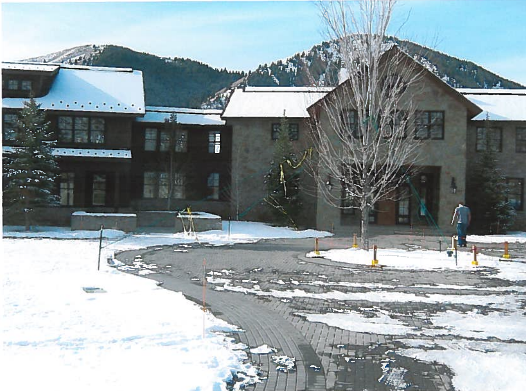
Example of pavement snowmelting (main entrance to house)
