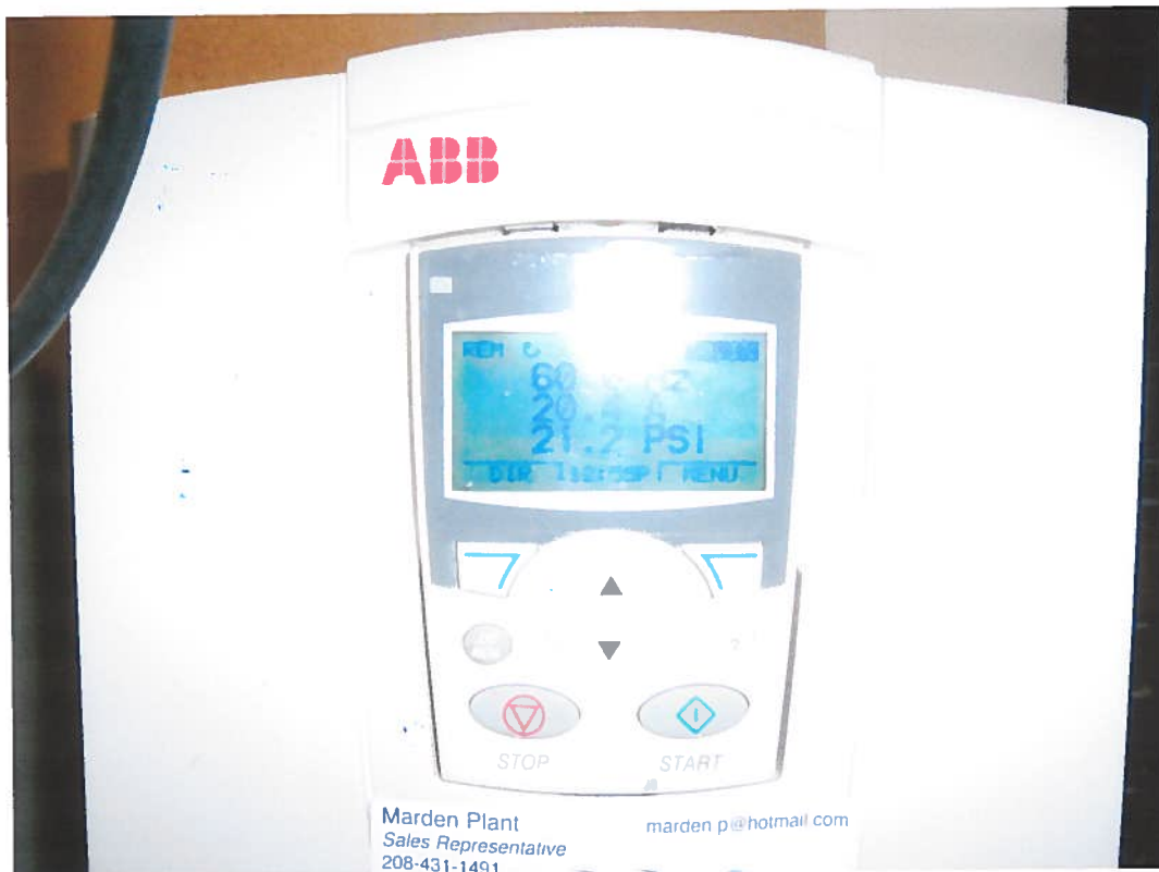
Variable-frequency drive
