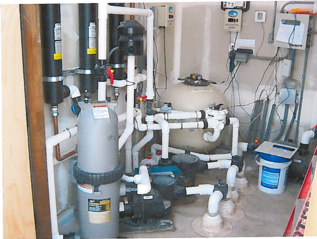
Heat exchanger system for pool and spa
