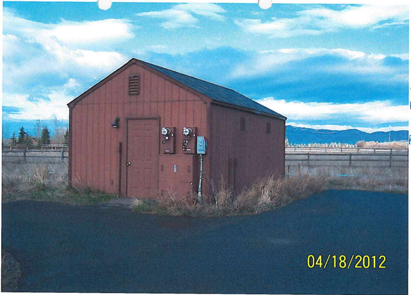
Pump House located on Parcel F lot
