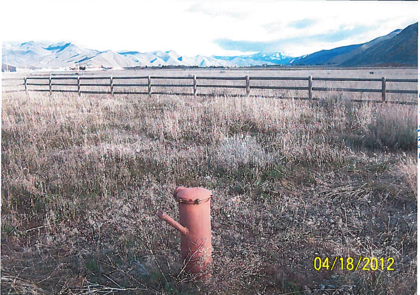
POD: North Well D002366 2 1/2" casing 29" above ground level
