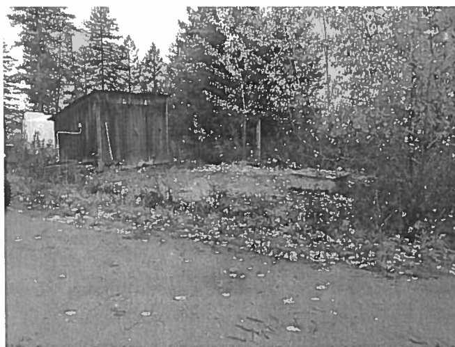
30,000-gallon concrete grade reservoir
