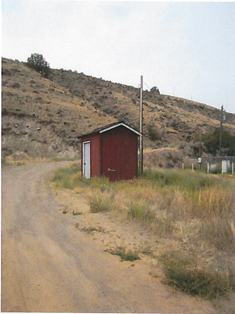
Location of the northern booster pump at the base of Galena Grade
