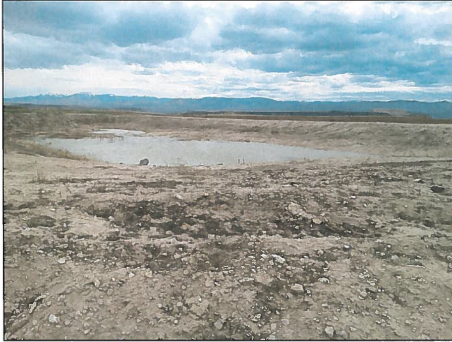
Figure 3: Stabilization pond with approximate storage capacity of 3 acre-feet.
