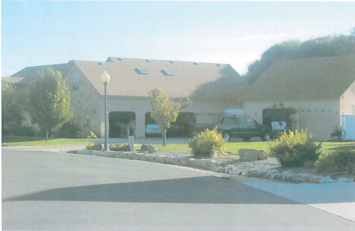
POU - picture of one of the 7 homes constructed in the subdivision.
