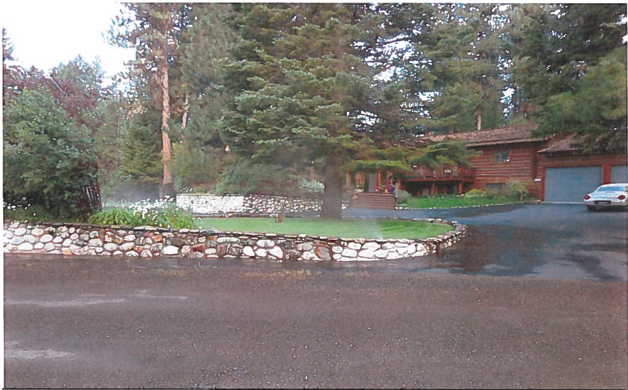
Place of Use: View westerly of one of the eight homes served by the Mile High Estates Subdivision water system. The pop-up rotary and spray sprinklers as shown in this photo, are typical of the individual pressurized irrigation systems serving each home.
