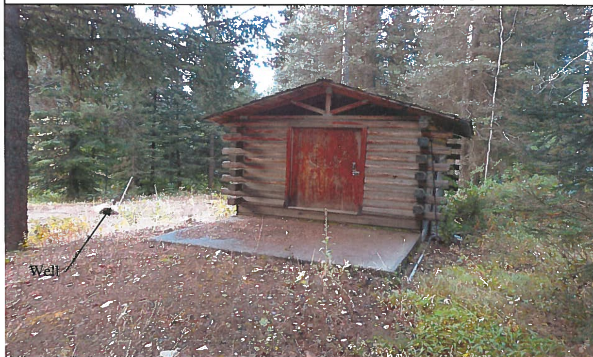
View southerly of the log pump house. The ground water well is shown near the pump house.
