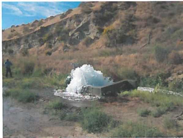
Pump discharge into lower canal – measurement of canal/pump flow taken to right of discharge. Return flow measurement taken to the left.
