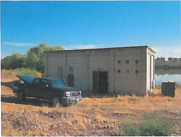
Pumphouse looking east.
