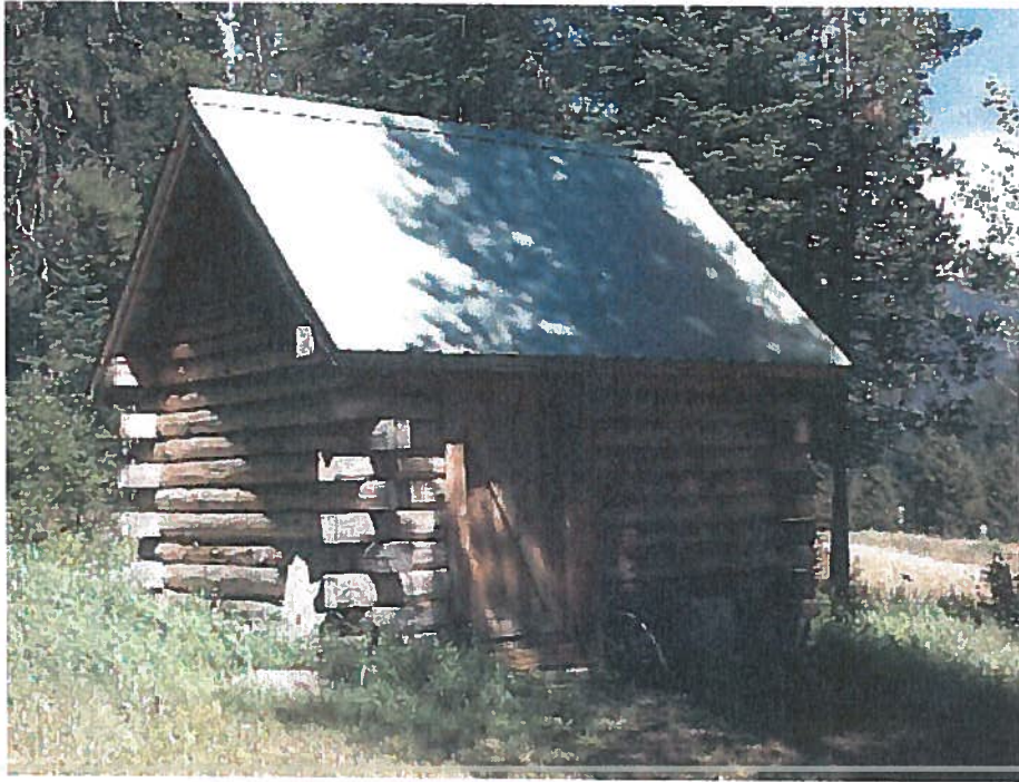
3. New wood-log powerhouse.
