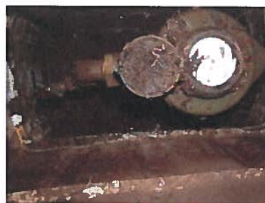
Vault with sample tap and flow meter
